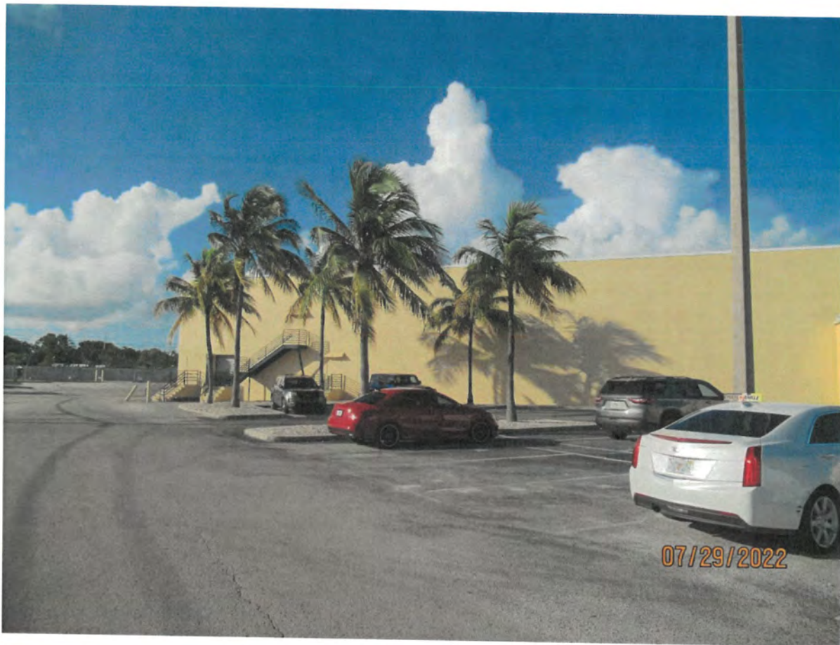
Photo showing existing conditions of rear parking area.
