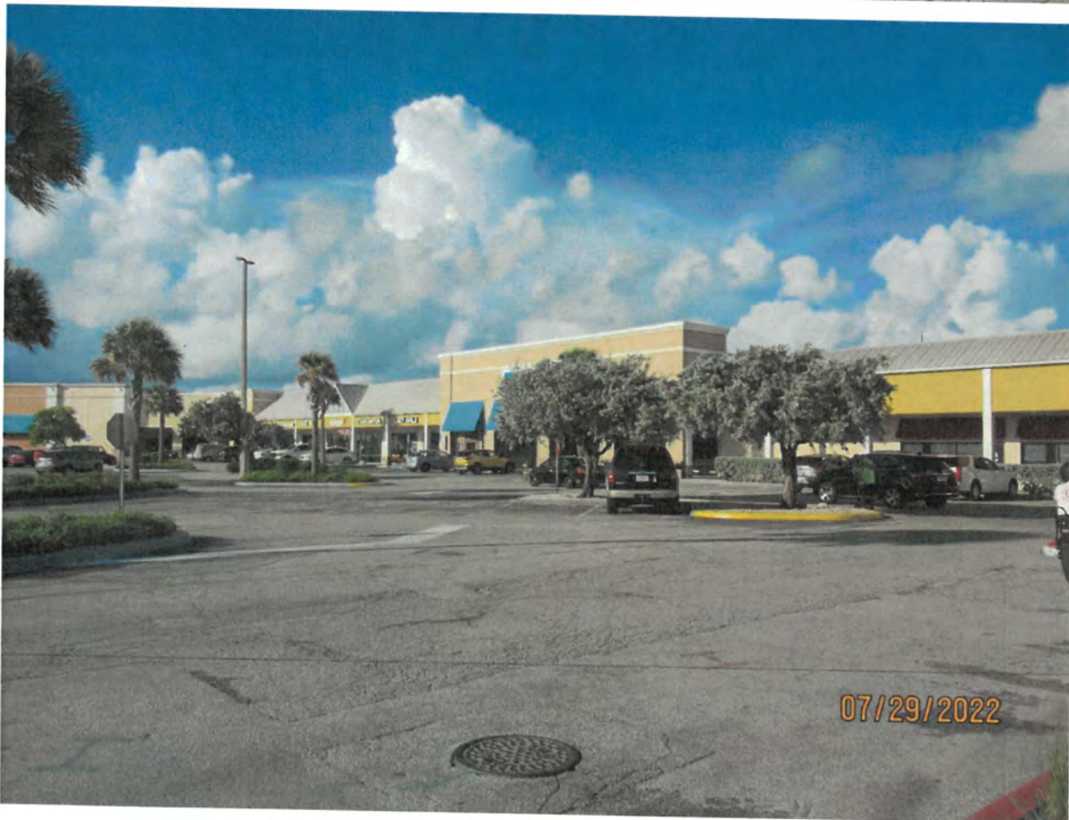
Two photo showing existing conditions of interior parking area. Most existing trees and palms will be transplanted on site.
