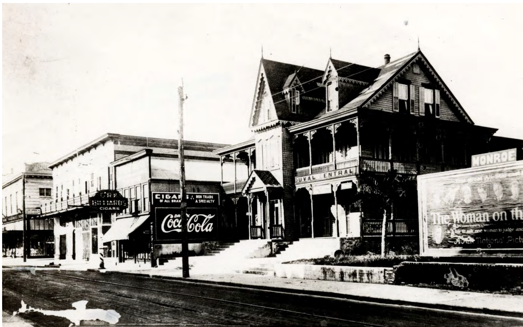
430 Duval Street circa 1924. Public Library was located on the Queen Anne building. After the building was demolished it was relocated across the street at 417 Duval Street. Monroe County Library.
