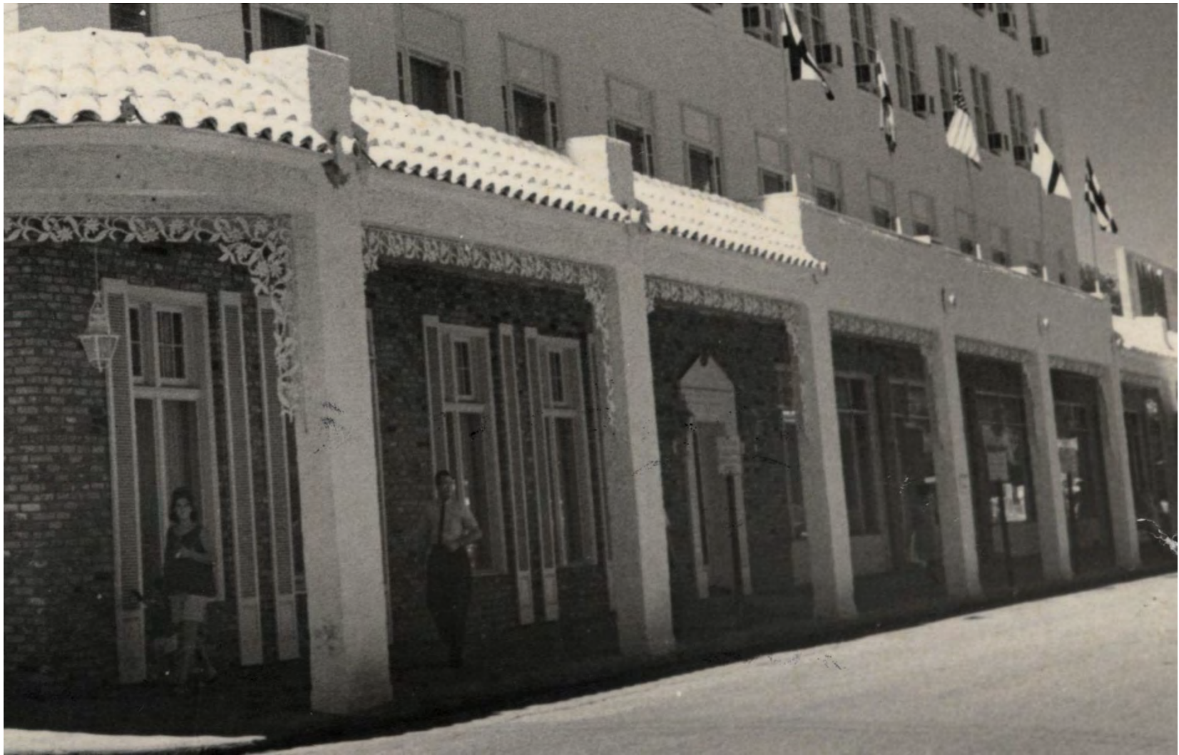
Detail of 1962 photograph. Monroe County Library.
