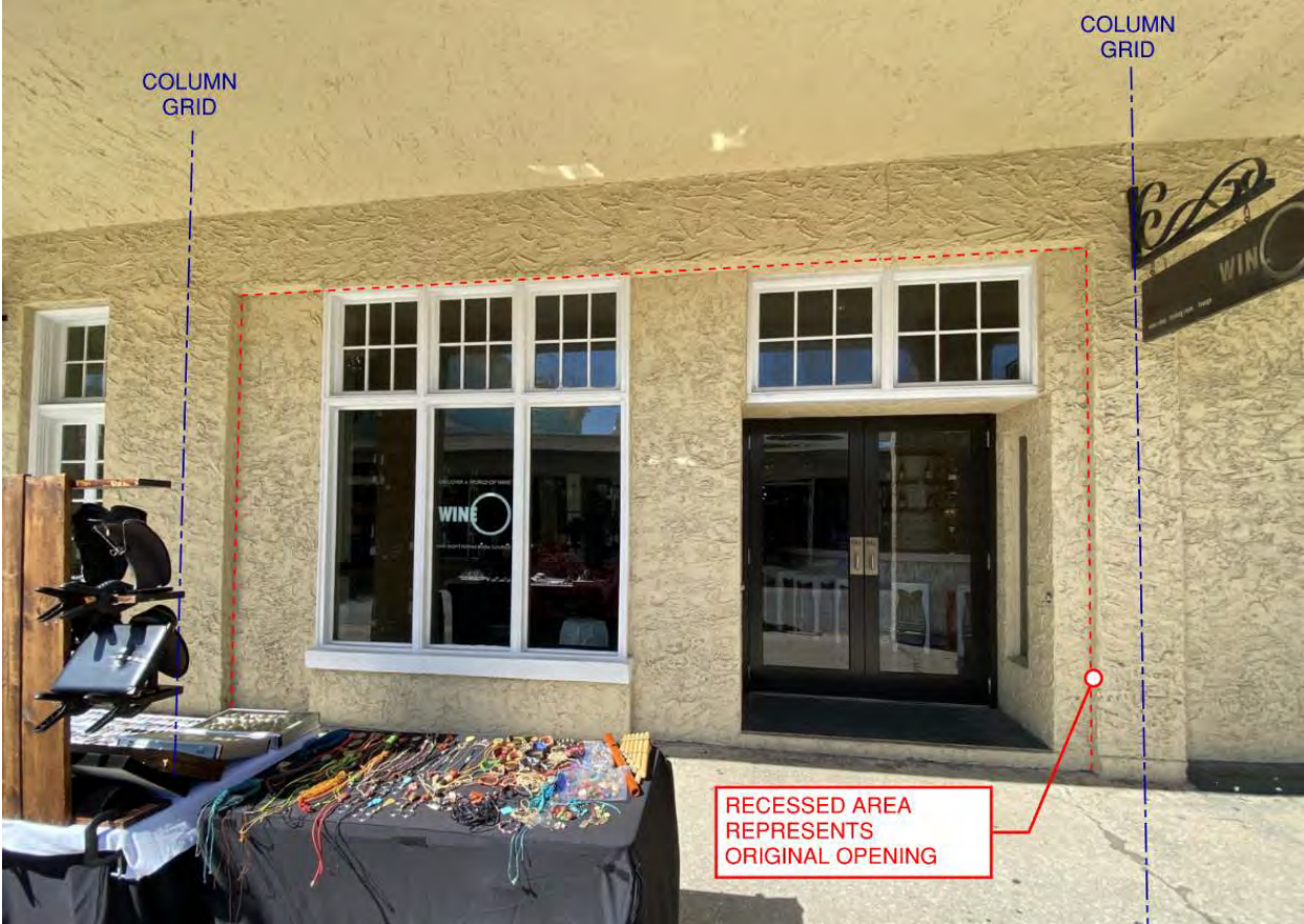
Bay 4 – existing conditions
