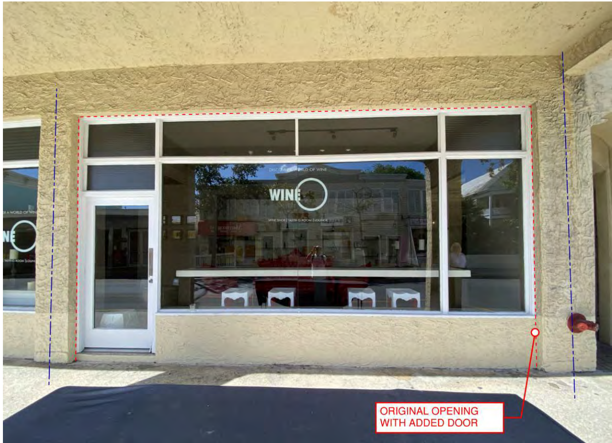
Bay 7 – existing conditions
