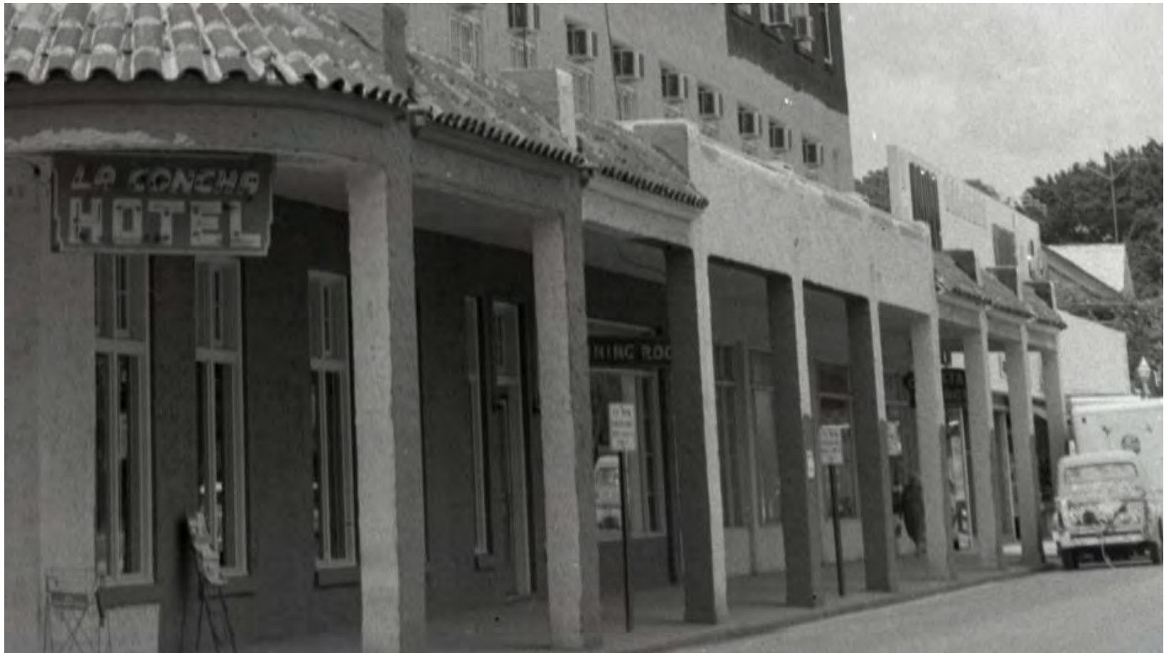
Detail of 1957 photograph. Monroe County Library.
