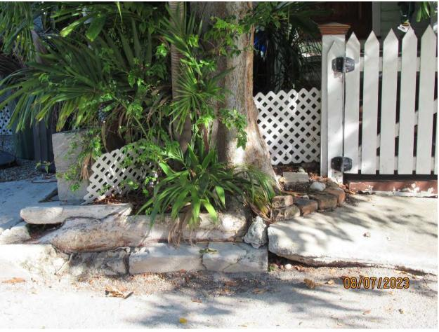
Photo showing base of tree and impacts to city sidewalk and curbing, views 2 & 3.
