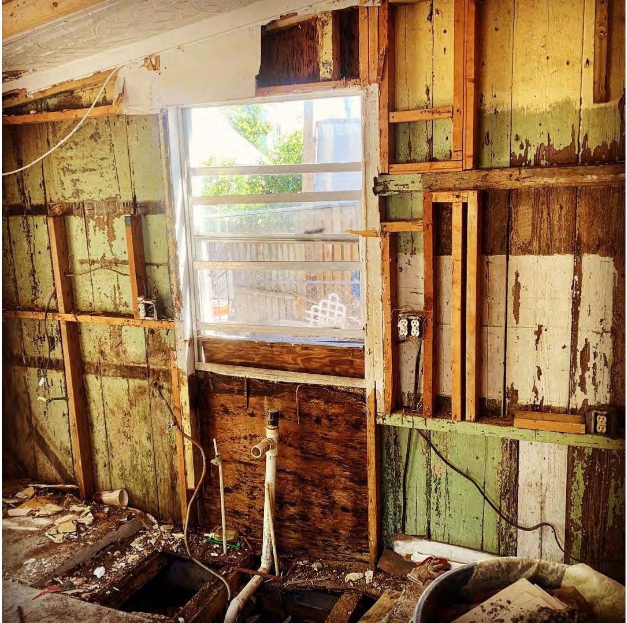
INSIDE OF REAR ADDITION (TO BE REMOVED)
