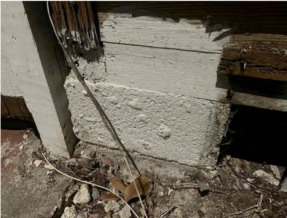
CONCRETE BLOCK FOUNDATIONS TYPICAL AT WEST SIDE ADDITION
