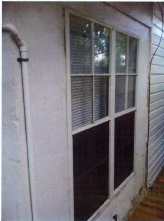
SOUTH WEST SIDE OF HOUSE EXISTING WINDOWS
