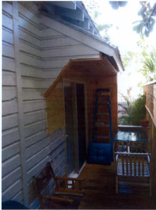
SOUTH WEST SIDE OF HOUSE LOOKING TOWARDS FRONT AREA WHERE SHED WAS REMOVED, ROOF STRUCTURE TO REMAIN
