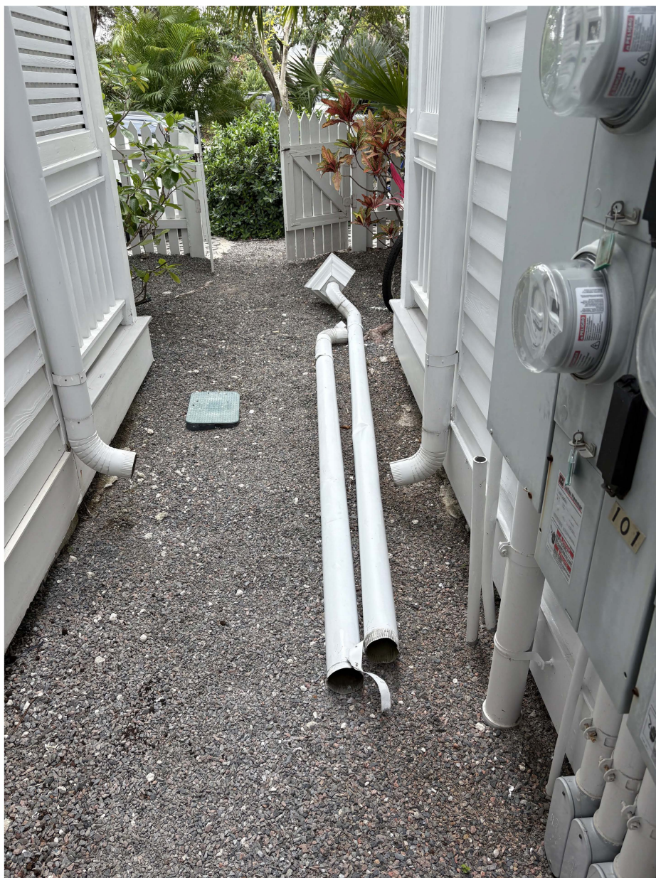
Emailed photo of fallen drainpipes
