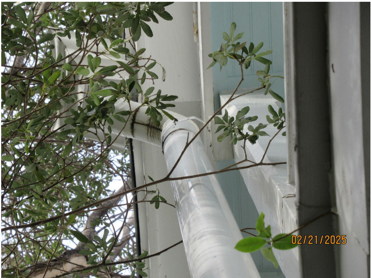
Photo looking at the drainpipe disconnecting from the railing and photo looking into canopy
