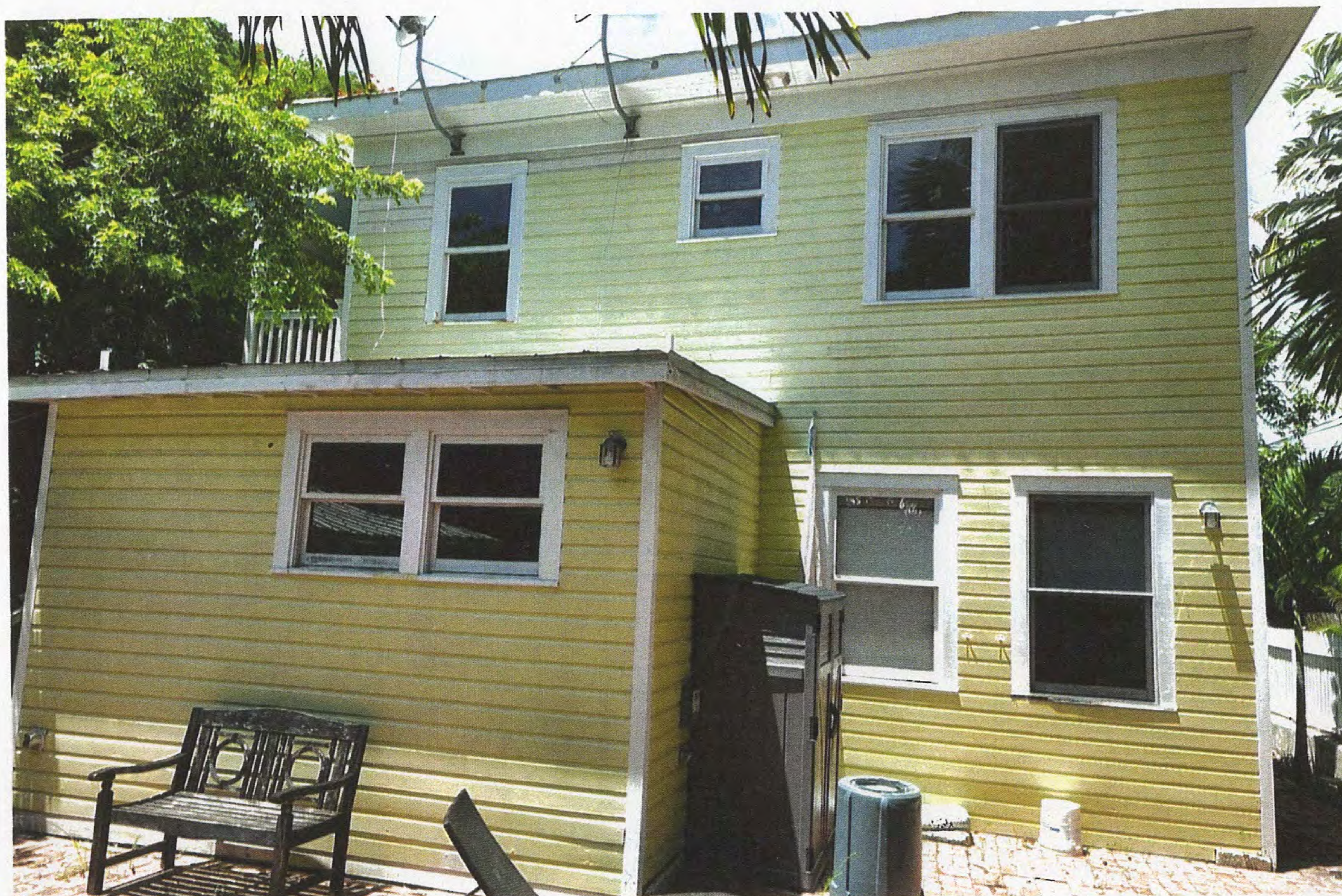
Rear view showing kitchen protrusion to be removed
