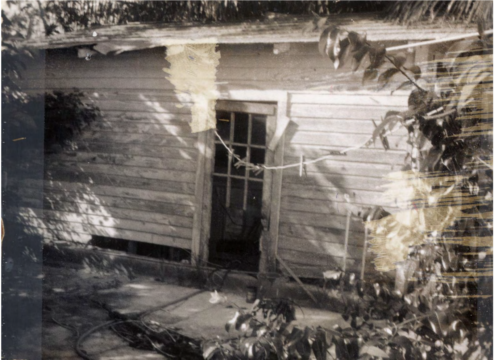
408 Virginia Street rear accessory structure in 1970. Monroe County Library.
