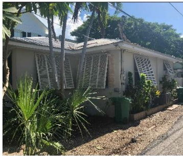
5 PHOTO OF 520 GRINNELL NORTH EXTERIOR ELEVATION
