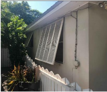
4 PHOTO OF 520 GRINNELL SOUTH EXTERIOR ELEVATION
