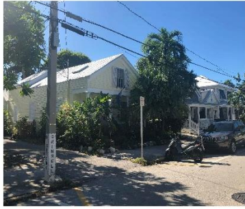
2 PHOTO OF ADJACENT PROPERTY TO THE NORTH
