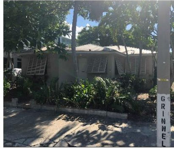
3 PHOTO OF 520 GRINNELL EAST EXTERIOR ELEVATION
