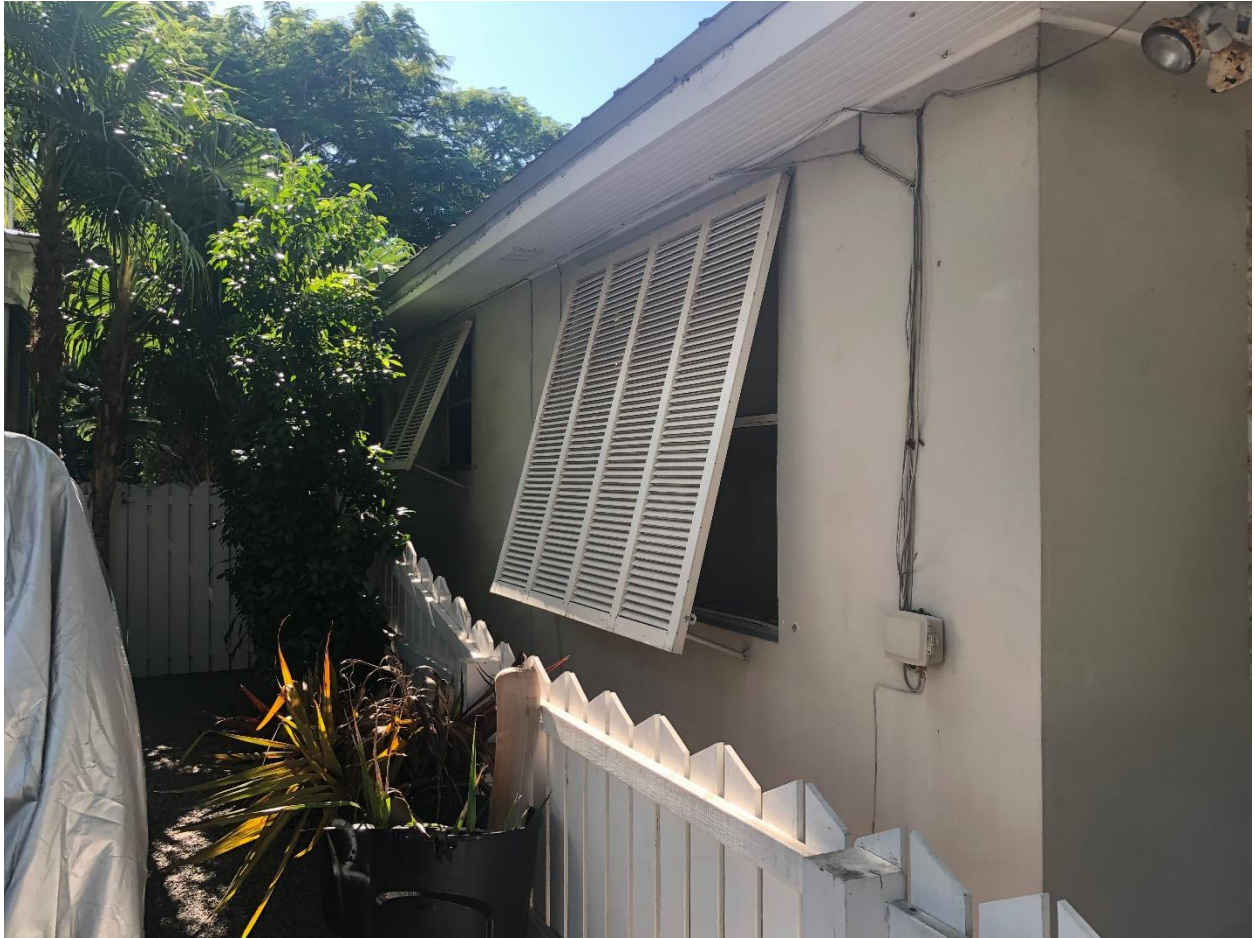
Photo of 520 Grinnell South Exterior Elevation.
