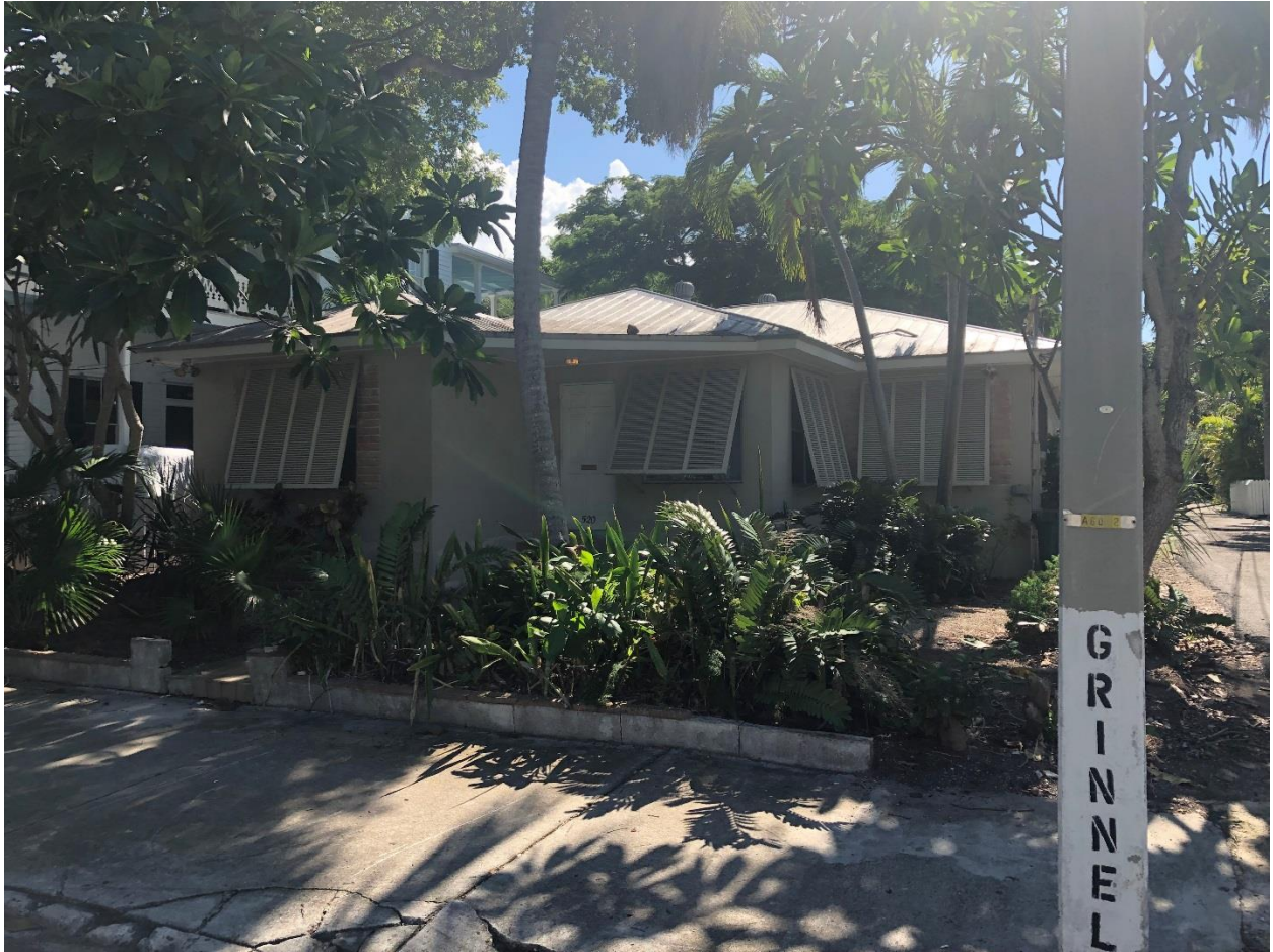
Photo of 520 Grinnell East Exterior Elevation.
