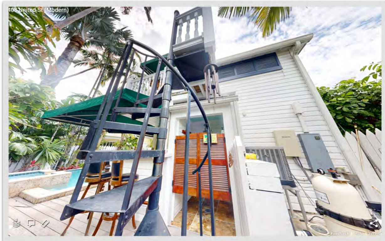
Rear spiral stairs (Egress for 2nd-floor bedroom)
