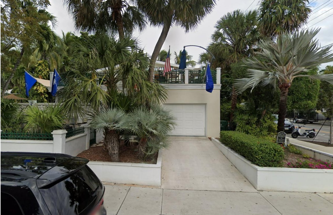
401 United Street showing metal railings on roof deck, built 1969.
