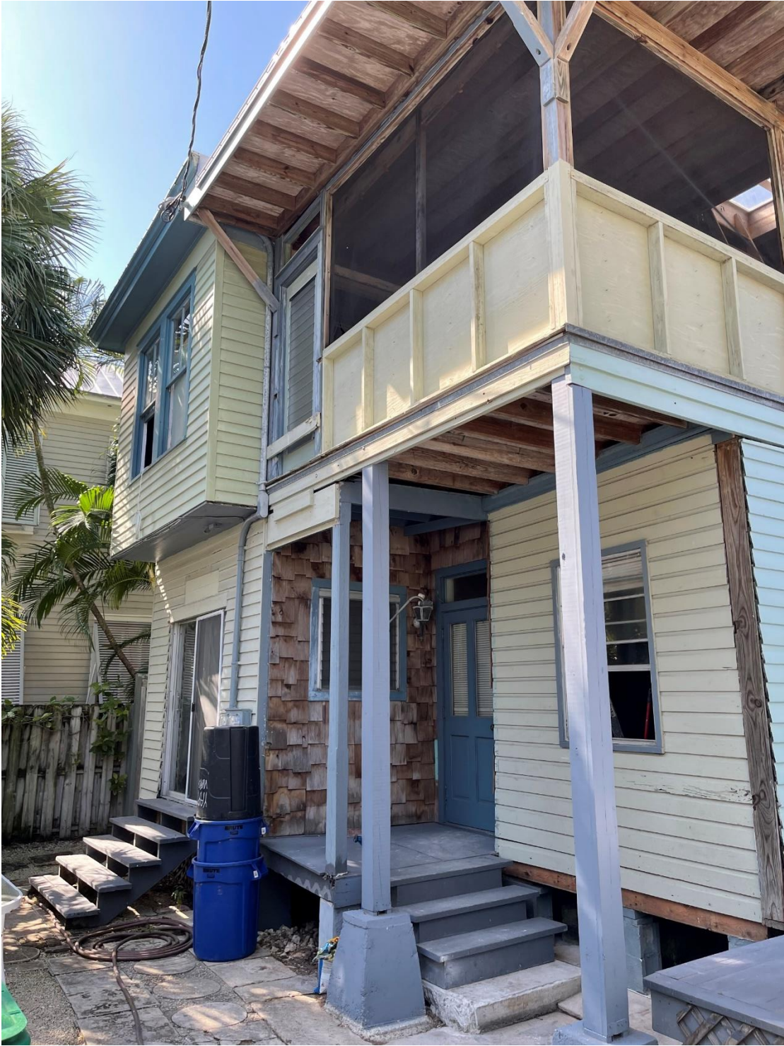
Rear of 1301 Whitehead before lifting and prior to renovation
