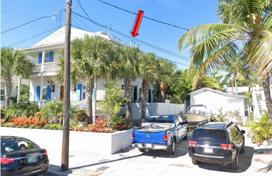
1315-1327 Whitehead Street showing cable railings, new construction 2015.
