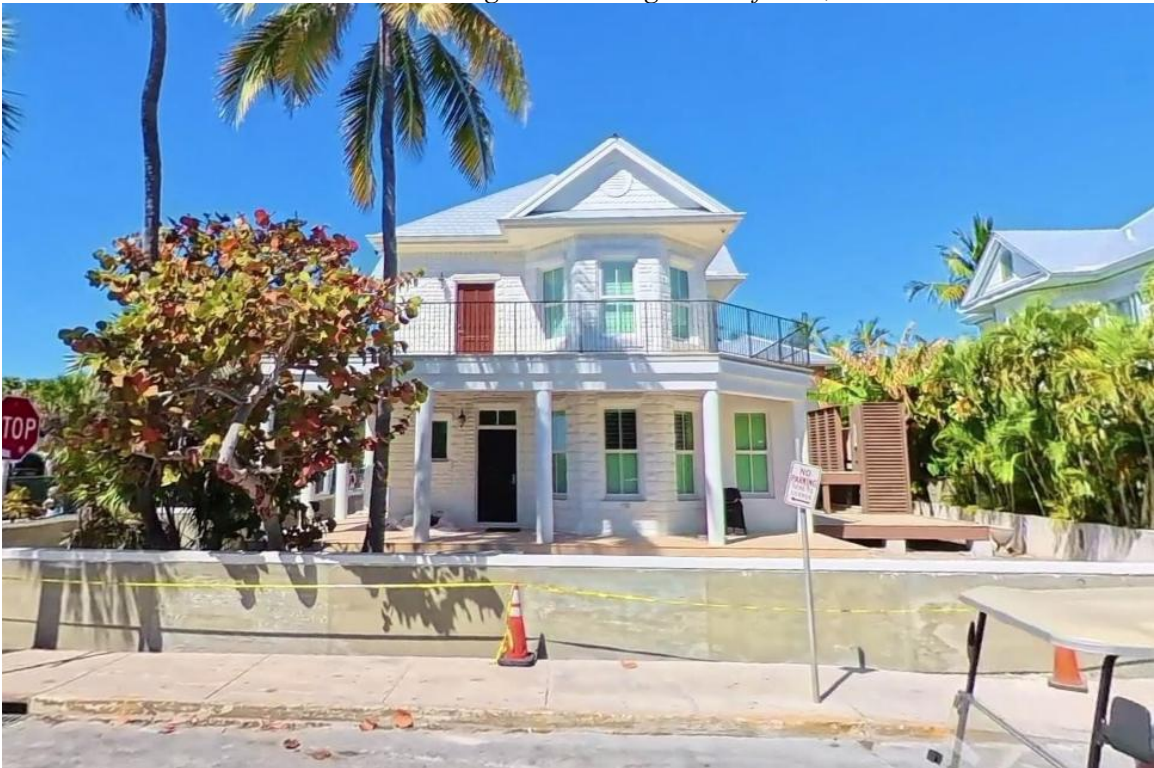
401 South Street showing metal railings, built circa 1912.
