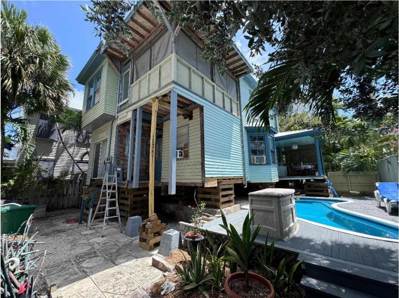
After Lift before North Wall demo
