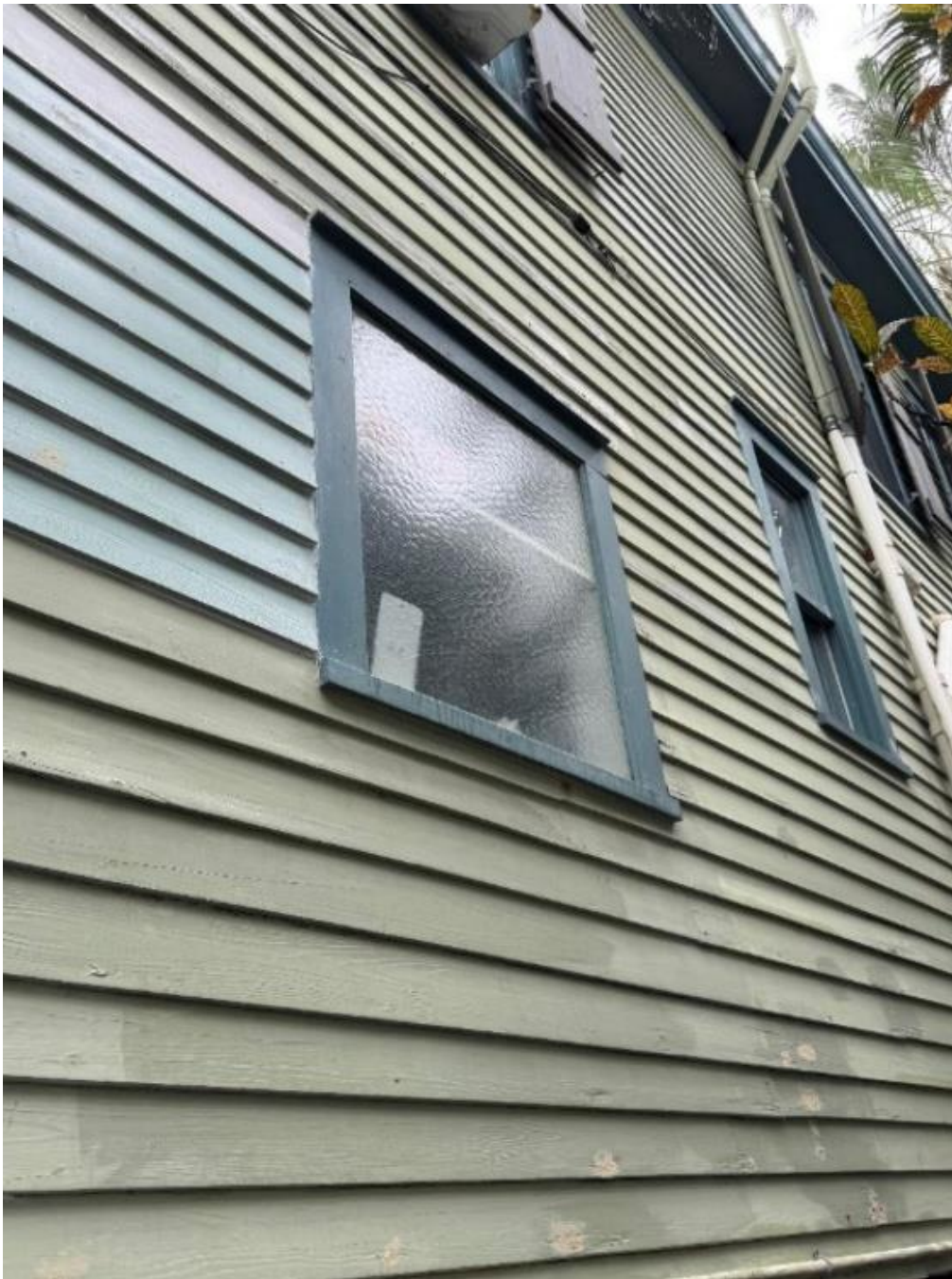
Southeast bedroom window, top is plexiglass
