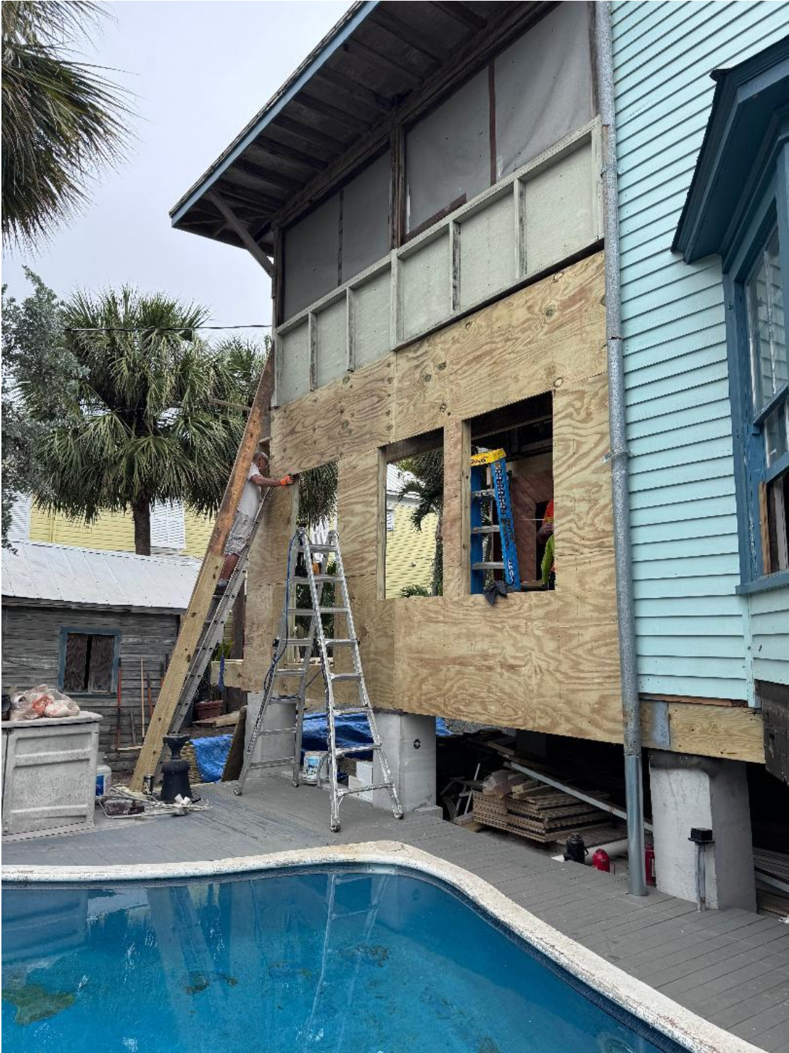
After Demo and Framing
