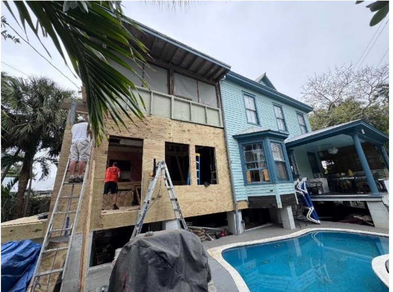
Northeast wall reframed with door and windows per plans
