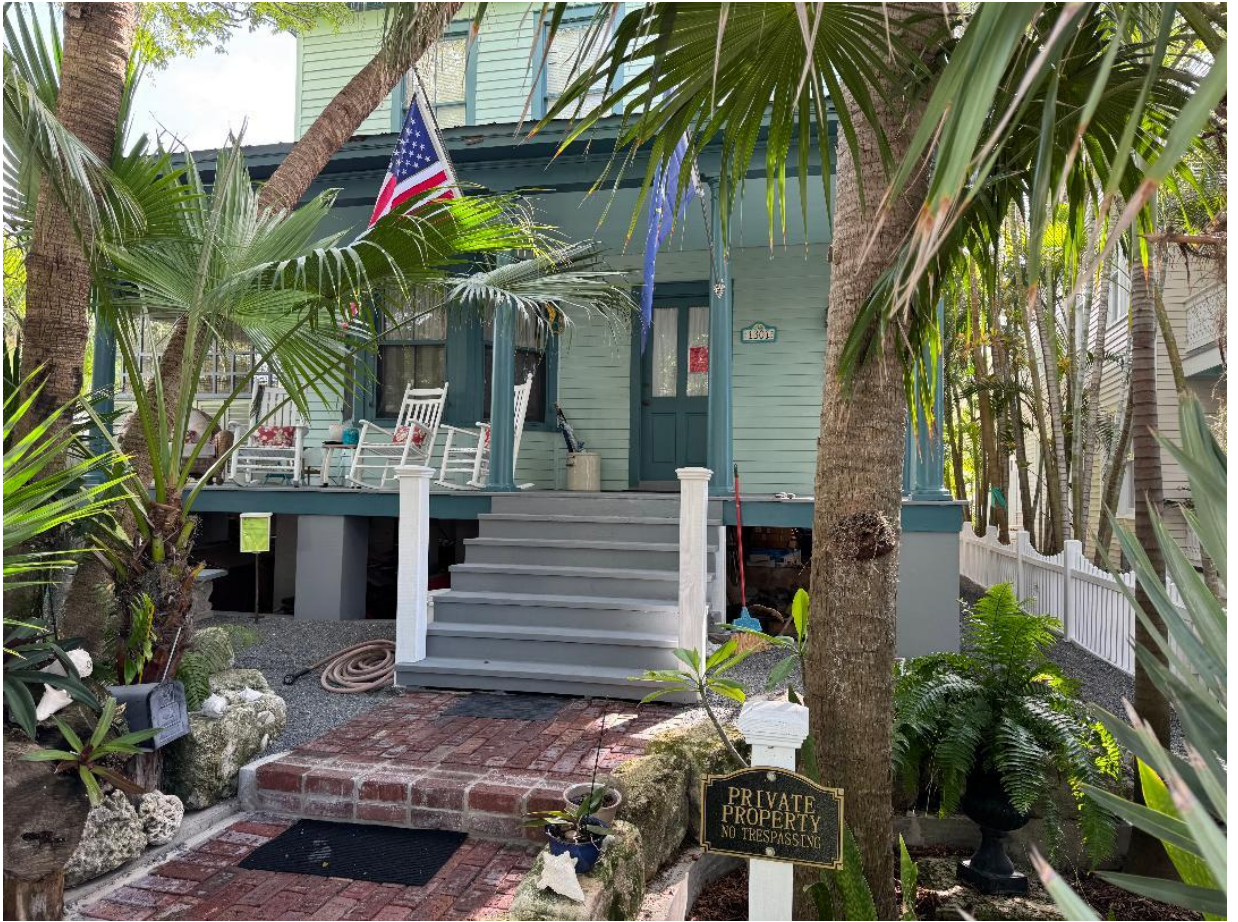
Current Front Entry of Home after lifting 3' 6"
