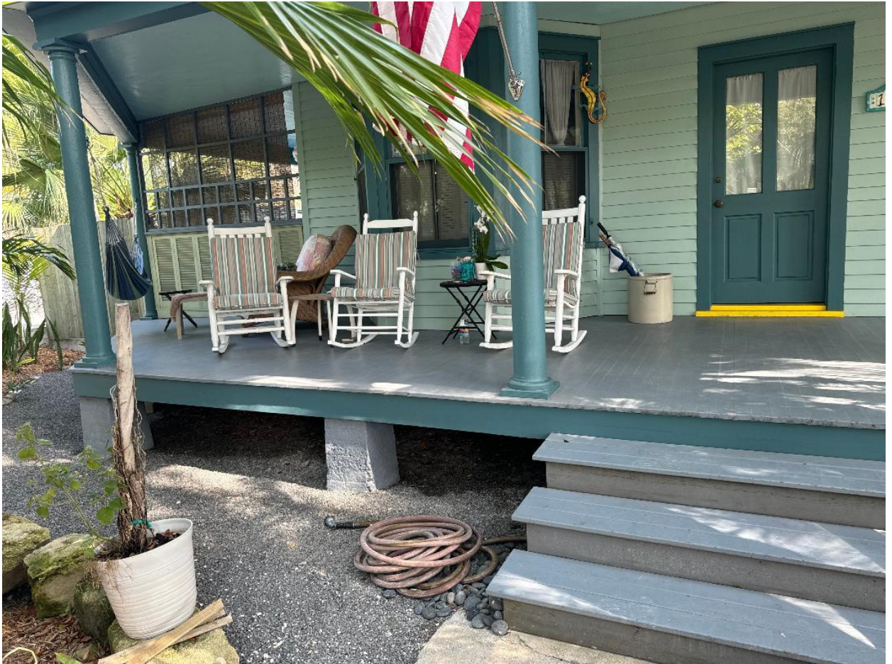
1301 Whitehead Prior to lifting home, prior to 15 May 2024
