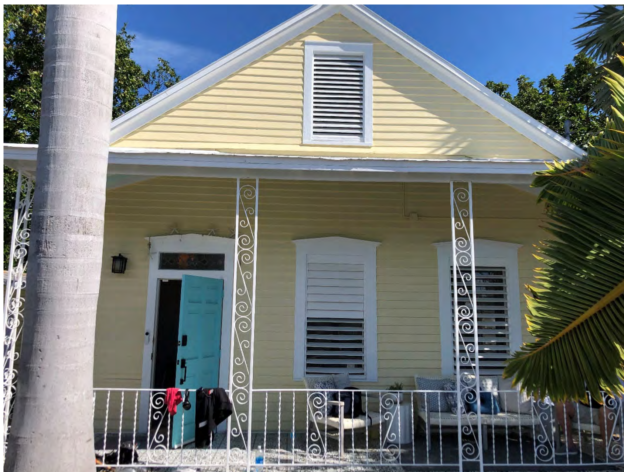
Façade / Street View
