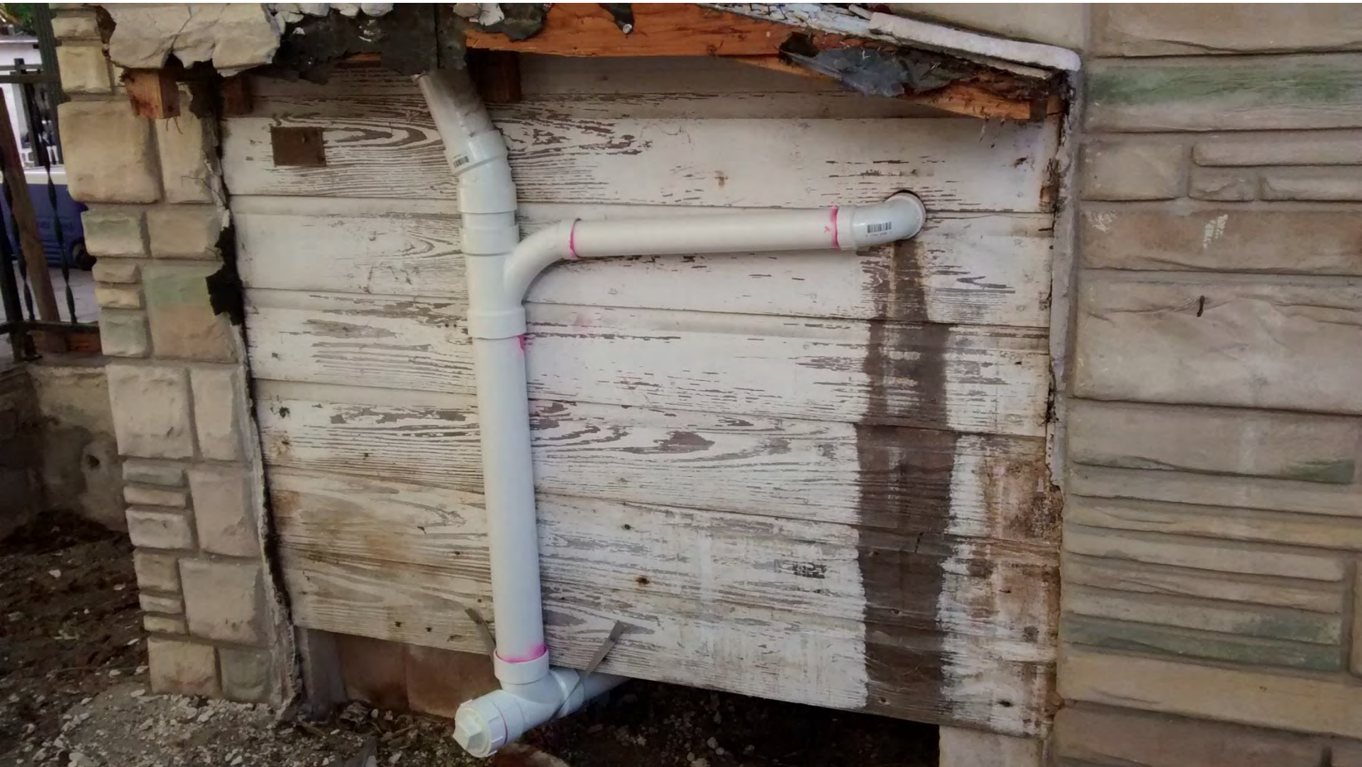
Wood novelty siding found underneath.
