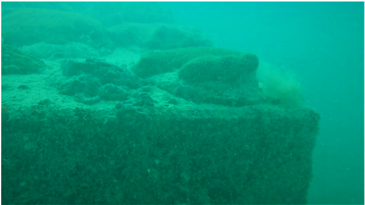
Photo 6. Typical seafloor conditions within the survey area adjacent to the existing pier. This is one of two large concrete blocks appx. 14' x 14' x 12" tall and supports a previous coral relocation project.
