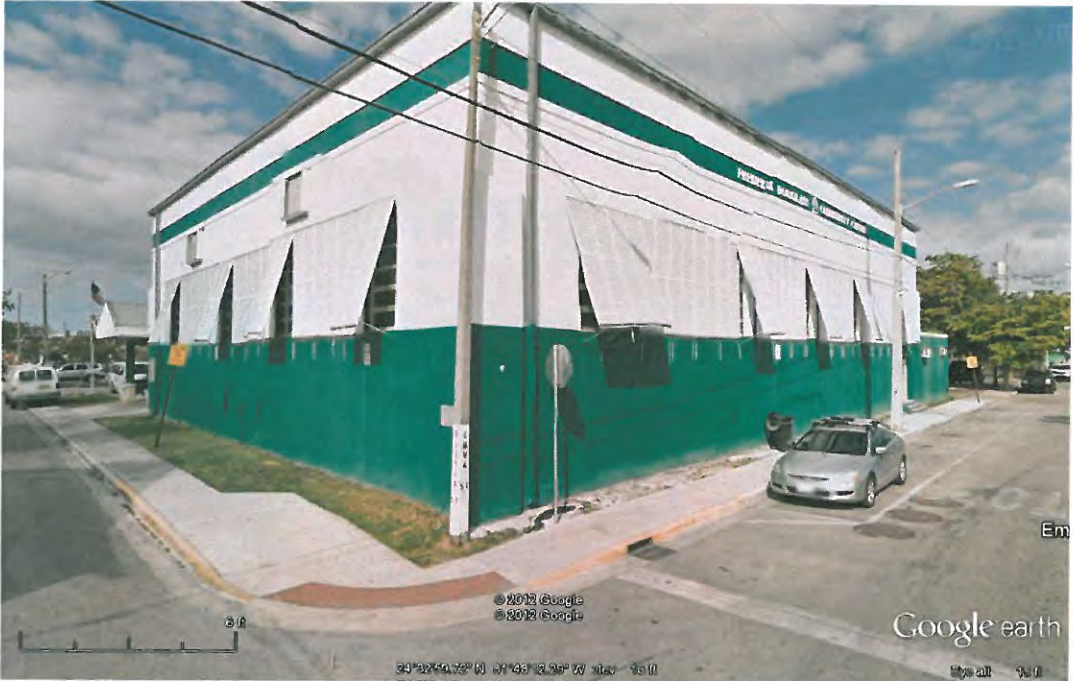
Northeast View of Building
