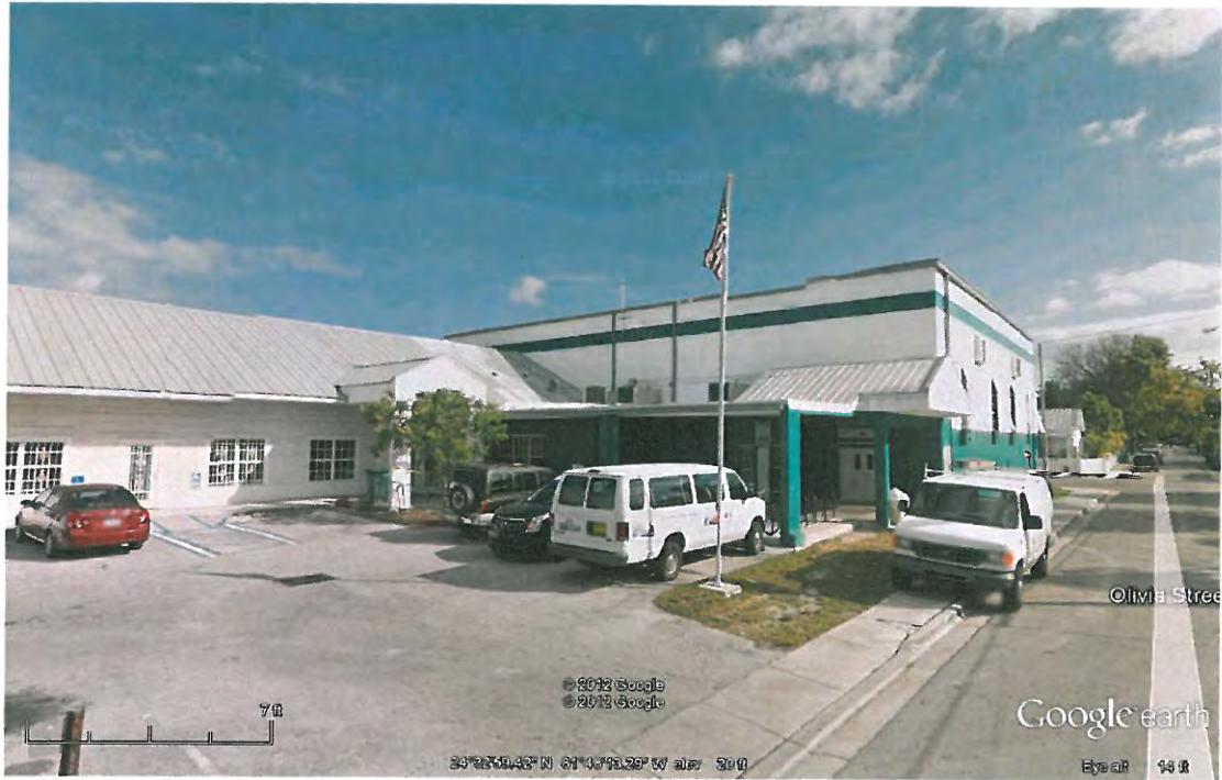
Southwest View of Building
