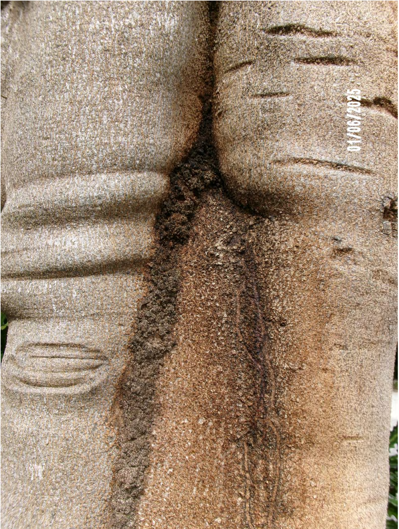
Termite mud trail in main trunk.
