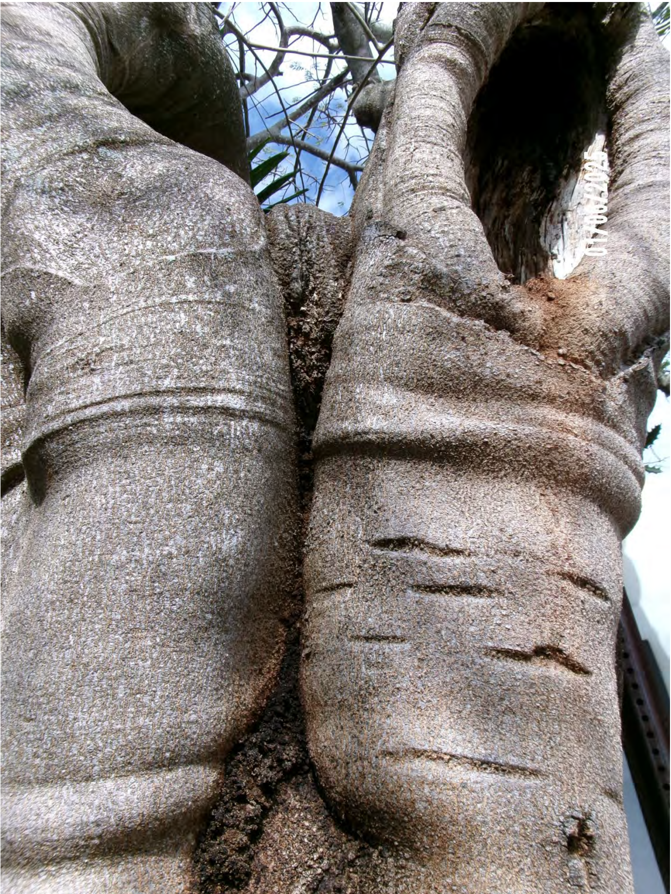
Close up of mud trail in the included bark area of the tree crotch.
