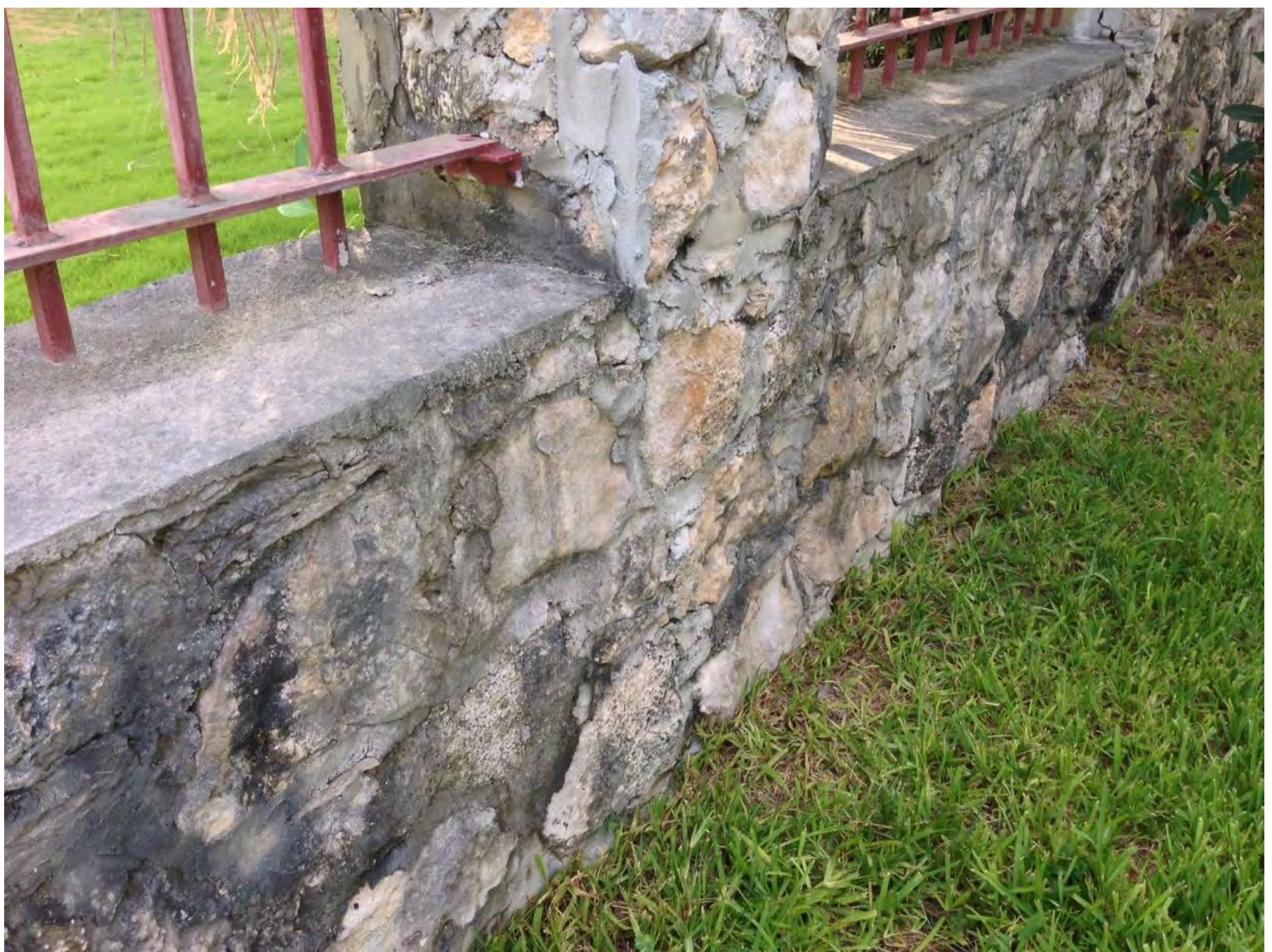
Portion of wall to be demolished.
