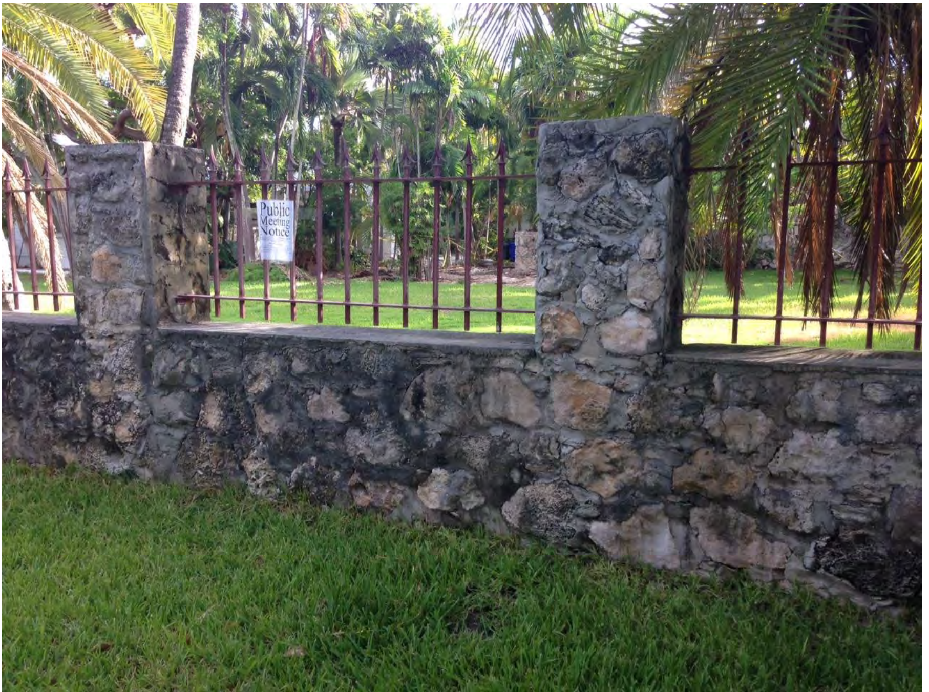
Portion of wall to be demolished. The left column will remain.
