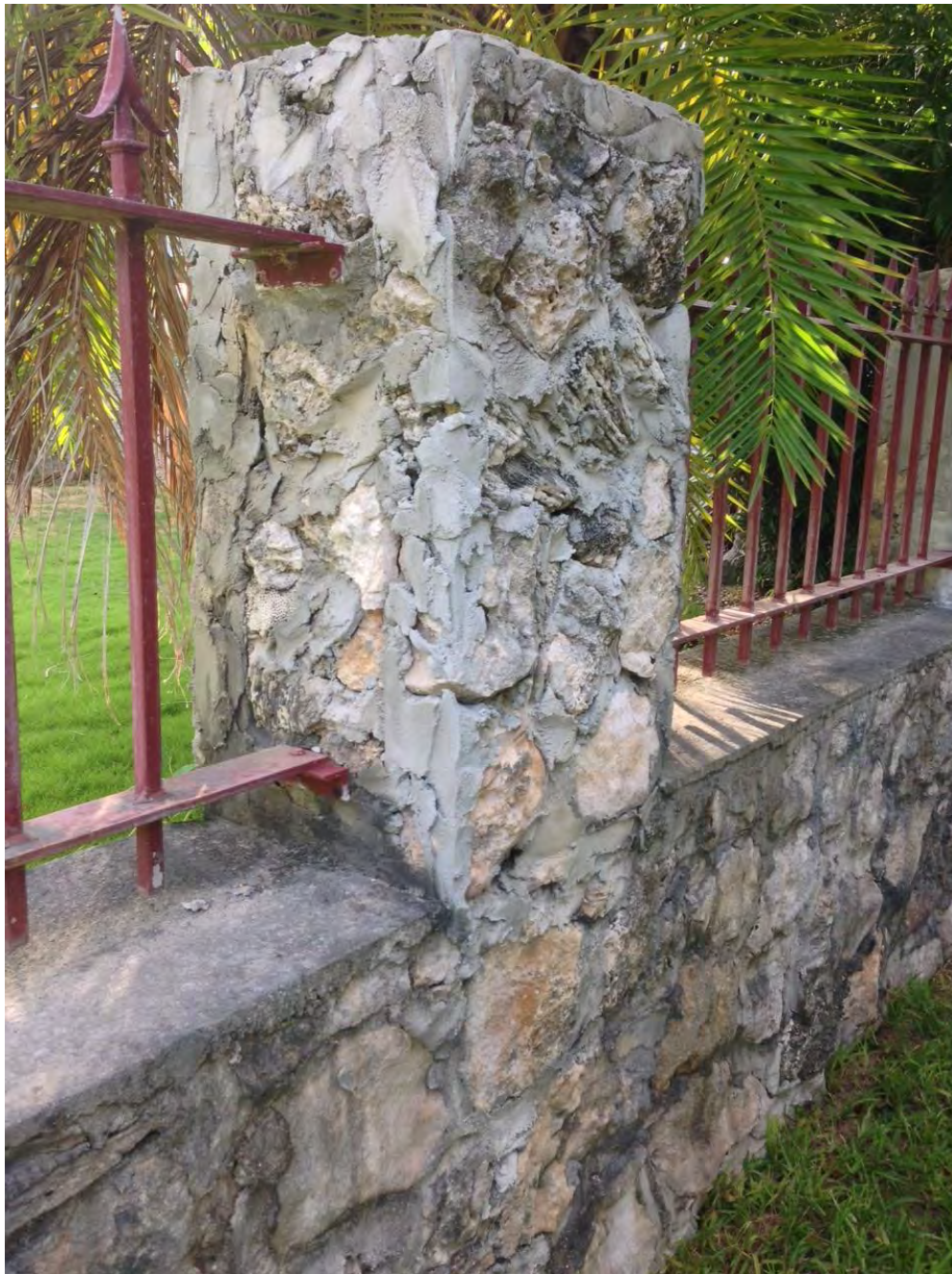
Portion of wall to be demolished.
