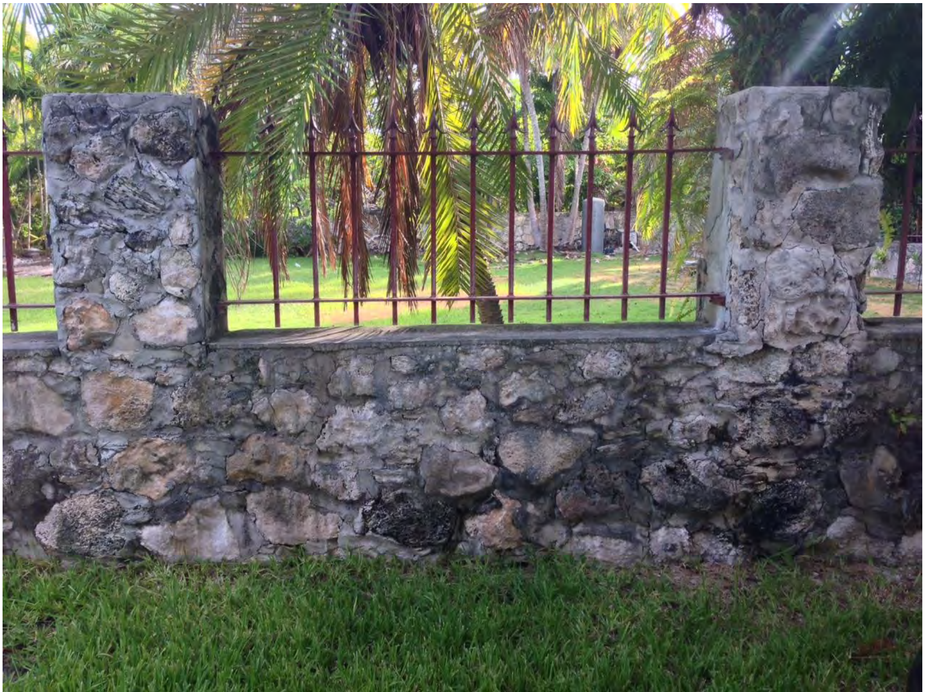
Portion of wall to be demolished. The right column will remain.
