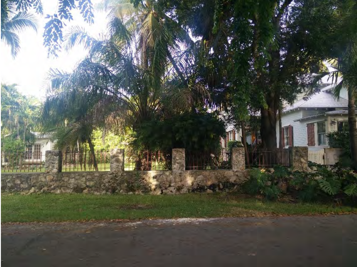
View of the historic wall surrounding the property on Whalton Street
