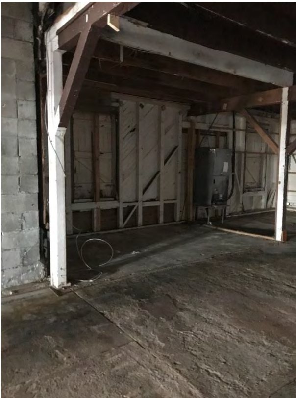
Charles Street structure rear wall adjacent to Smokin Tuna
