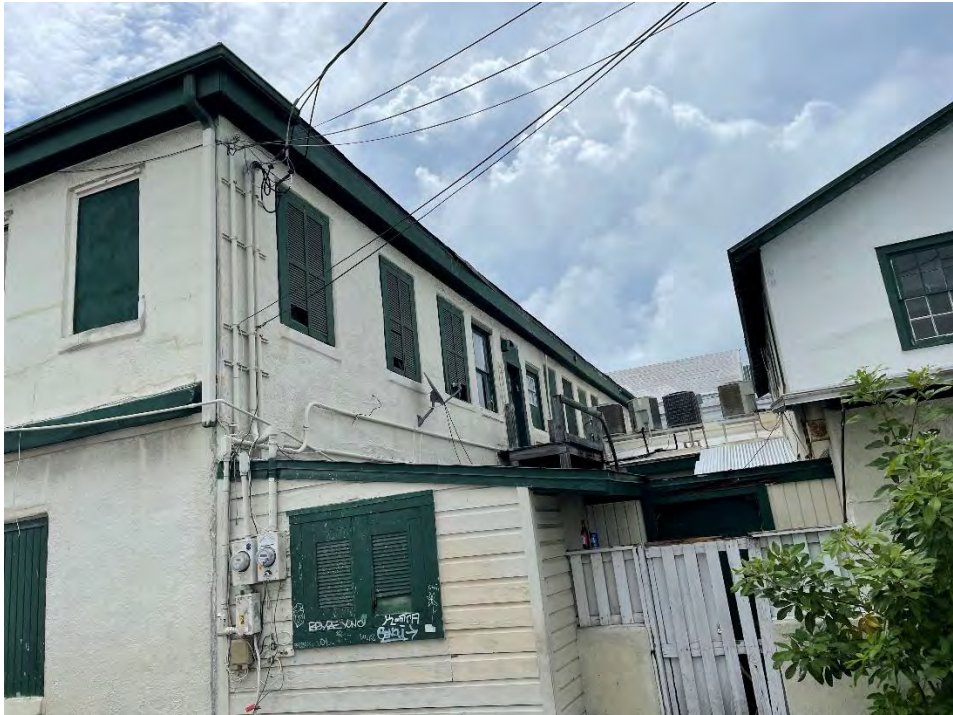
Rear of 210 Duval building
