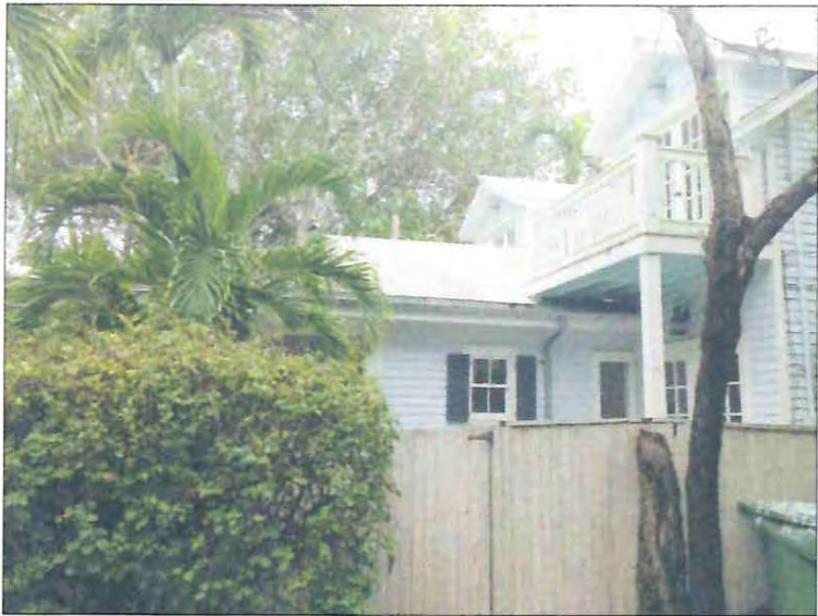
FIGURE 2 VIEW FROM JOHNSON LN
