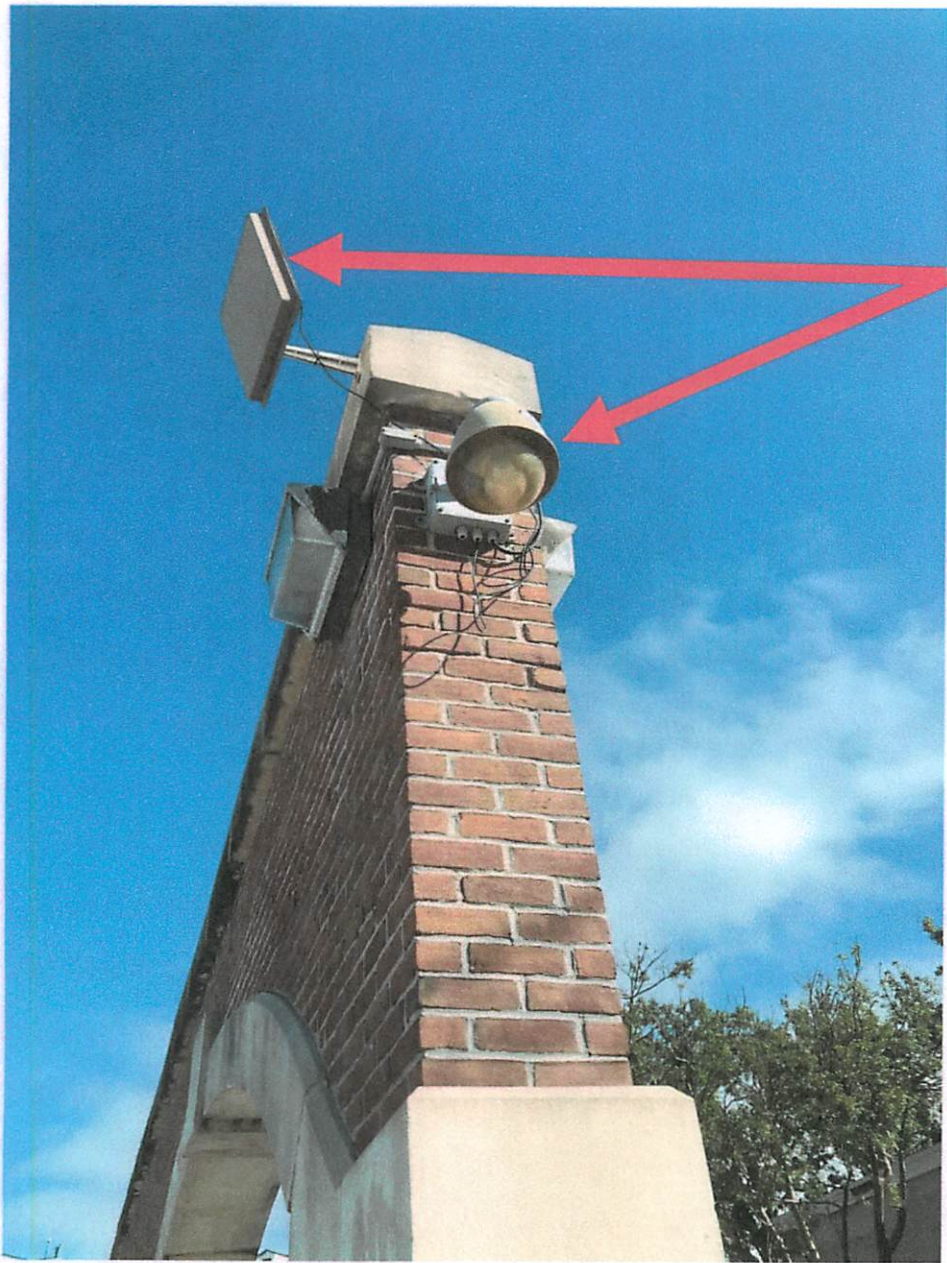
Old cameras/antennas on arches at Mallory
