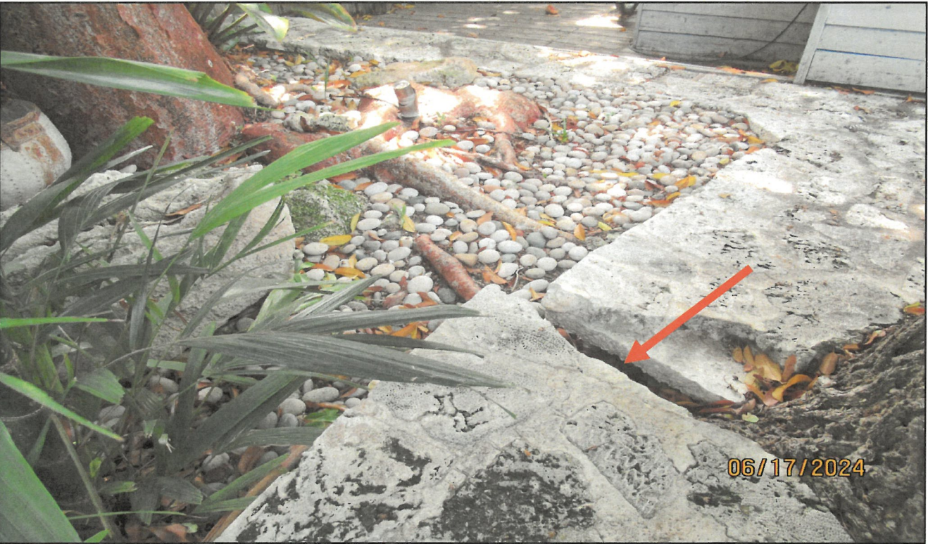
Alternate views of cracked sidewalks from expanding roots.
