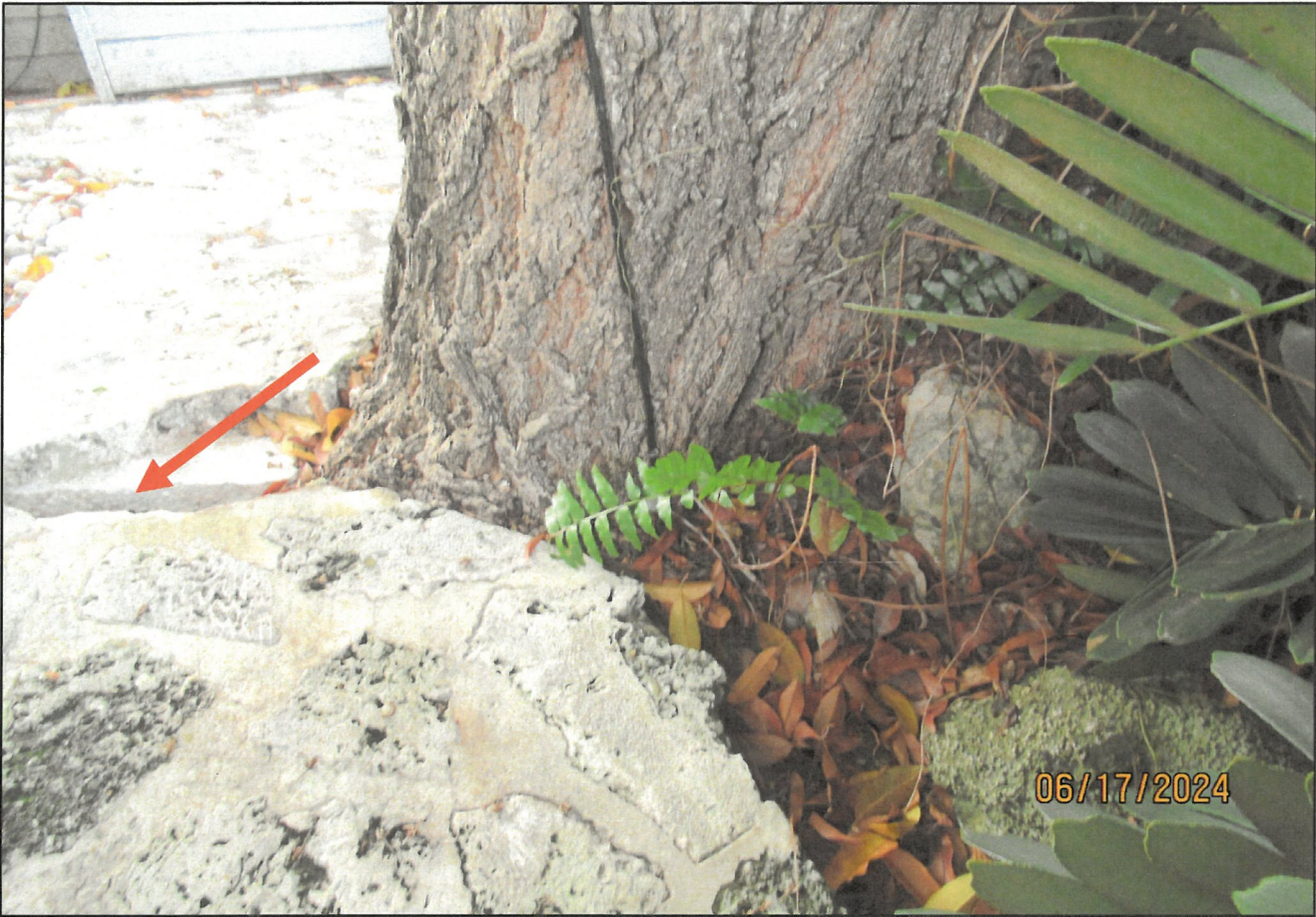
Alternate views of cracked sidewalks from expanding roots.
