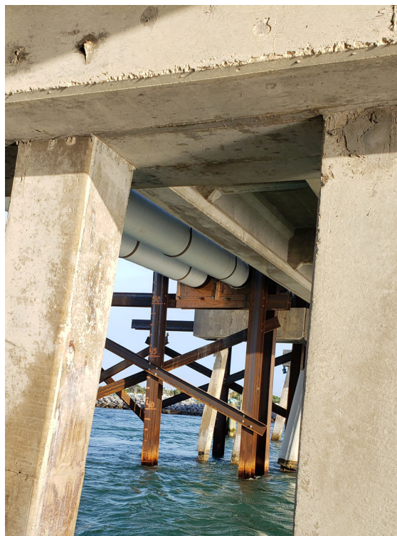
Figures 2. Side view of temporary stabilization.
