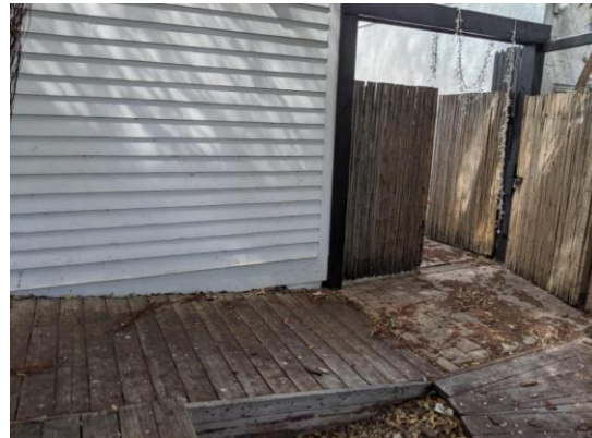
Rear yard ADA ramp
