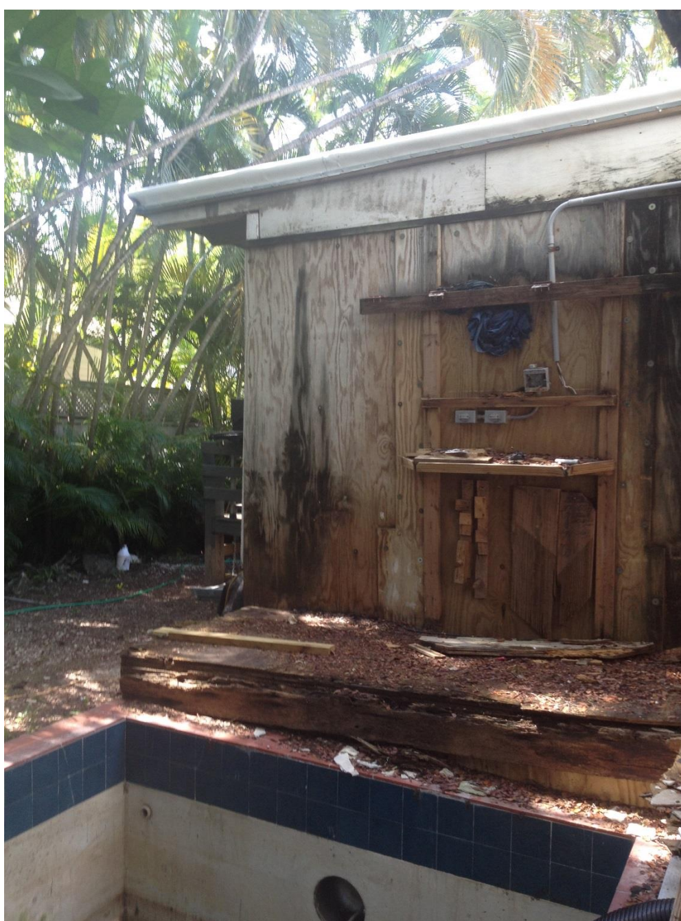
Rear of 818 Sawyers Lane
