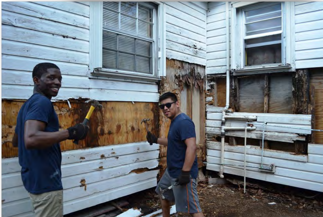
306 Truman Into repairs of the exterior siding, etc.
