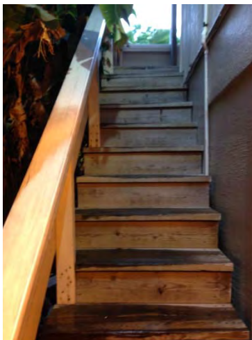
Photograph 1 showing the stairs to the second story addition.
