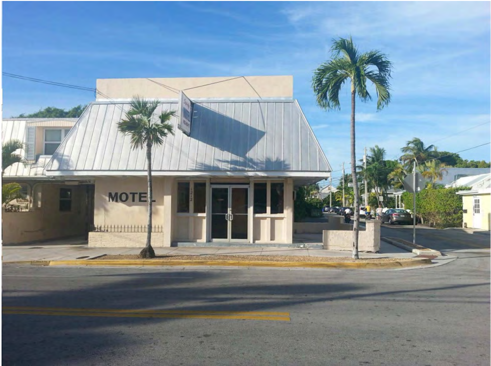
The Florida Motel today. Other than the parapet wall, all other character defining features are gone.
