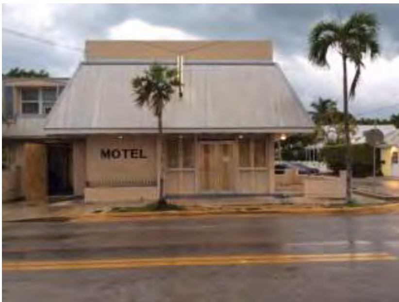
Exhibit B - Front façade on Simonton Street as seen today.
