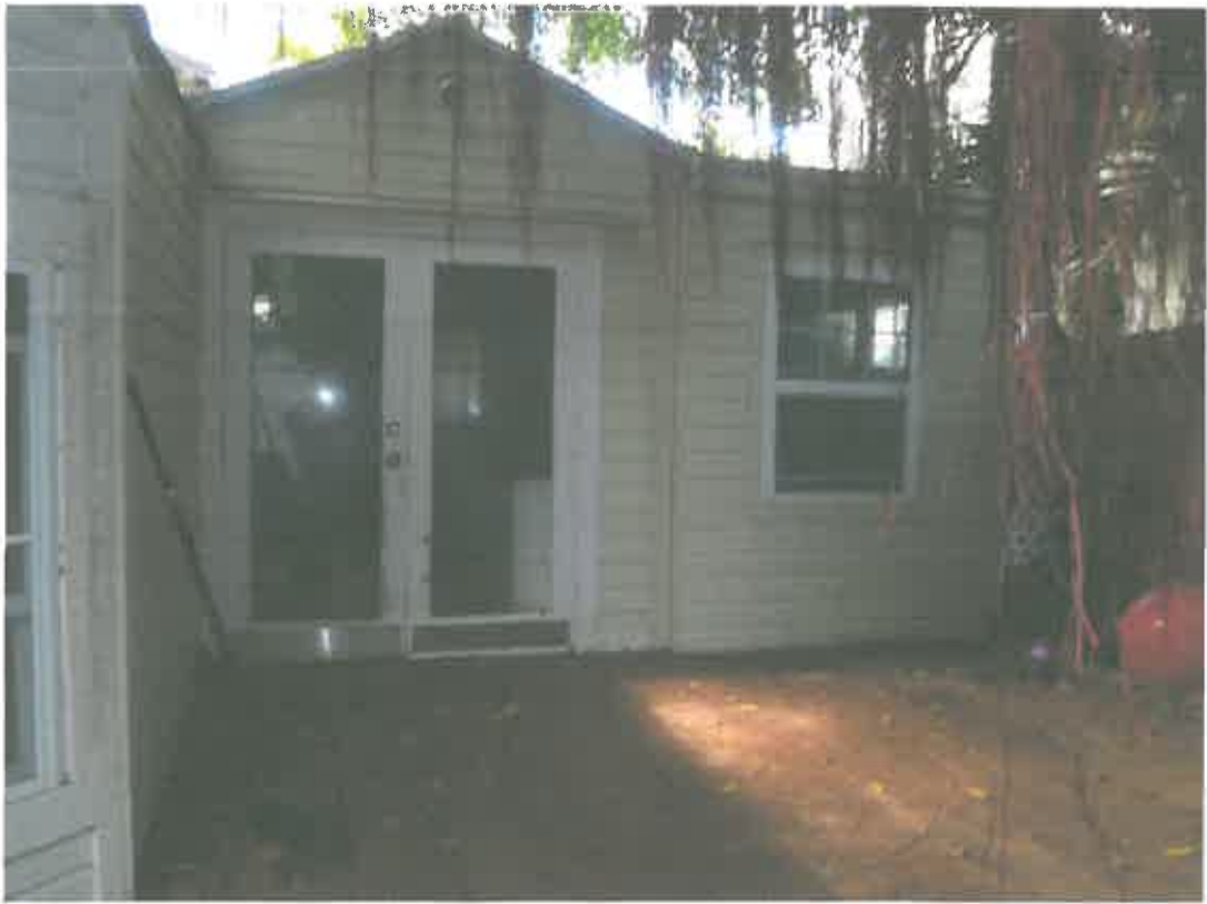
527 Margaret Street - Rear Yard
