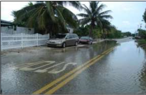
High-tide flooded road on Big Pine Key
