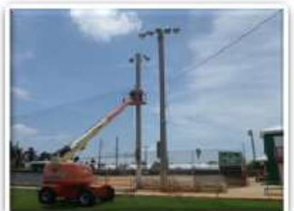
Key West ball field lighting retrofit
