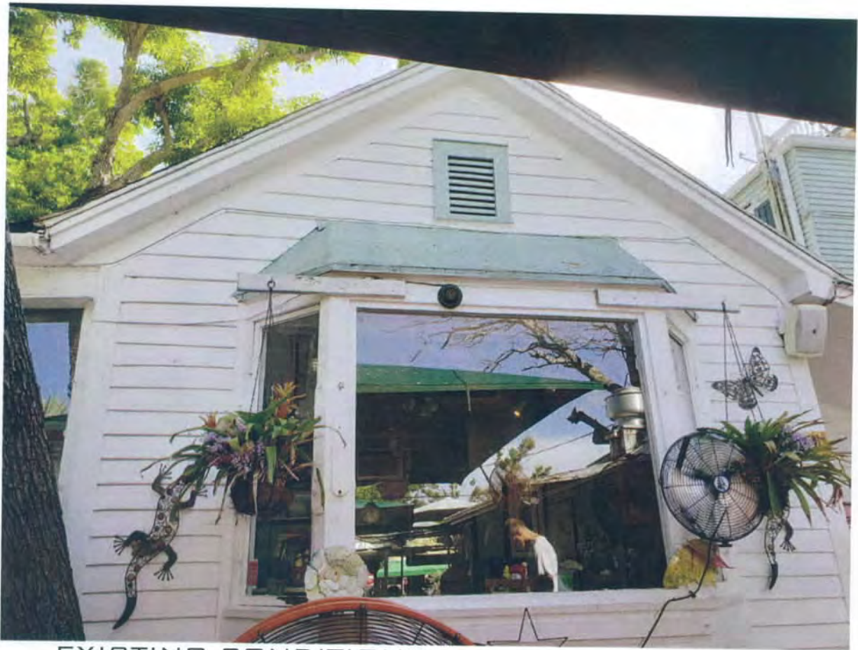
EXISTING CONDITIONS FRONT VIEW OF PROPOSED KITCHEN BUILDING
