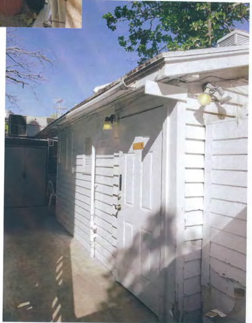
EXISTING CONDITIONS RIGHT SIDE OF PROPOSED KITCHEN BUILDING
