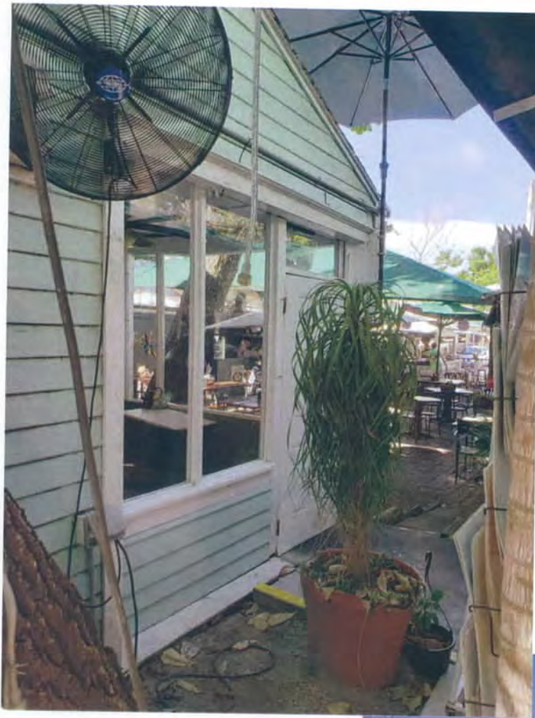
EXISTING CONDITIONS LEFT SIDE OF PROPOSED KITCHEN BUILDING
