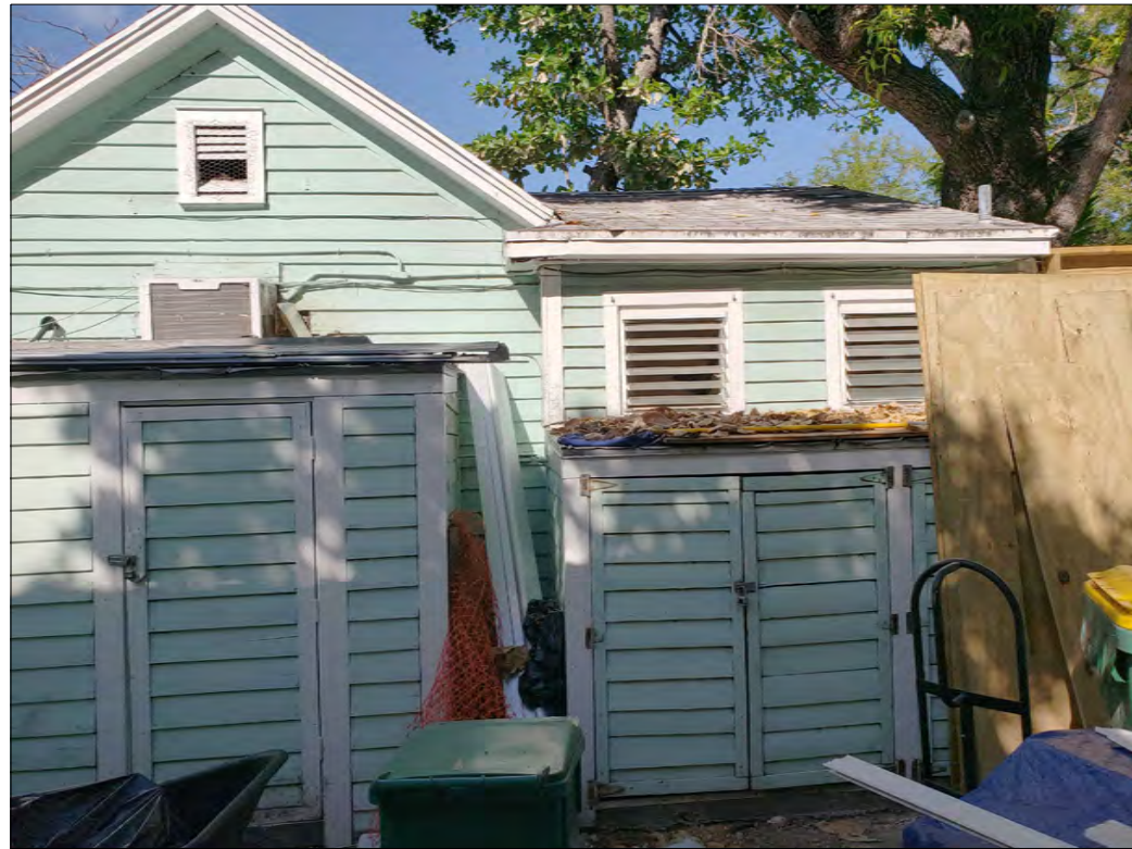
IMAGE 07, NEW KITCHEN ADDITION REAR SHEDS TO BE DEMOLISHED
