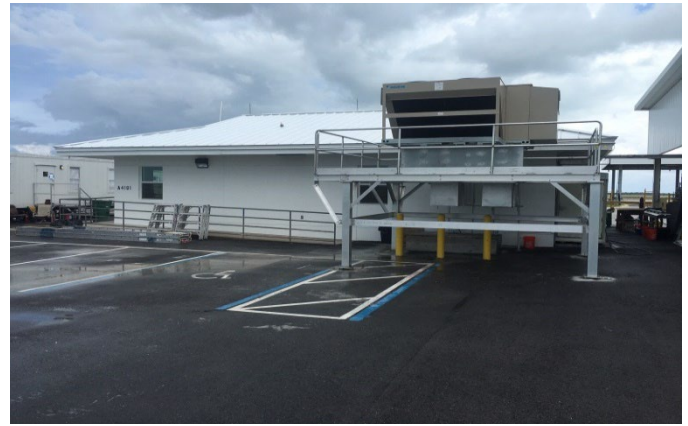
Design/Build Building A-4191 Boca Chica NAS, Key West
