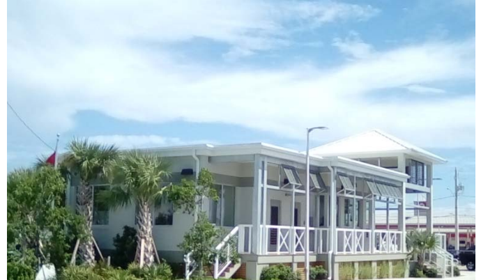
Dockmaster/Transient Restrooms, Garrison Bight, Key West
