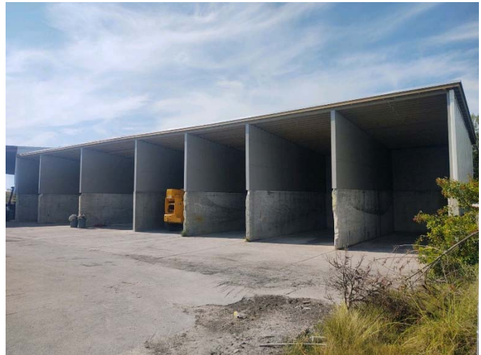
Long Key Transfer Station - Long Key, FL
