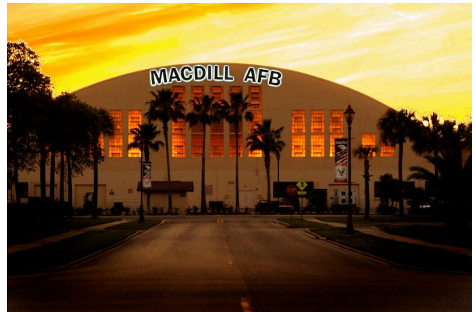
Design/Build Correct Commercial CNS Power Feed
