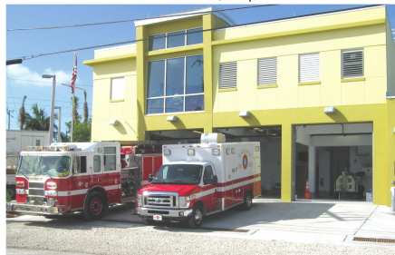
Conch Key Fire Station
