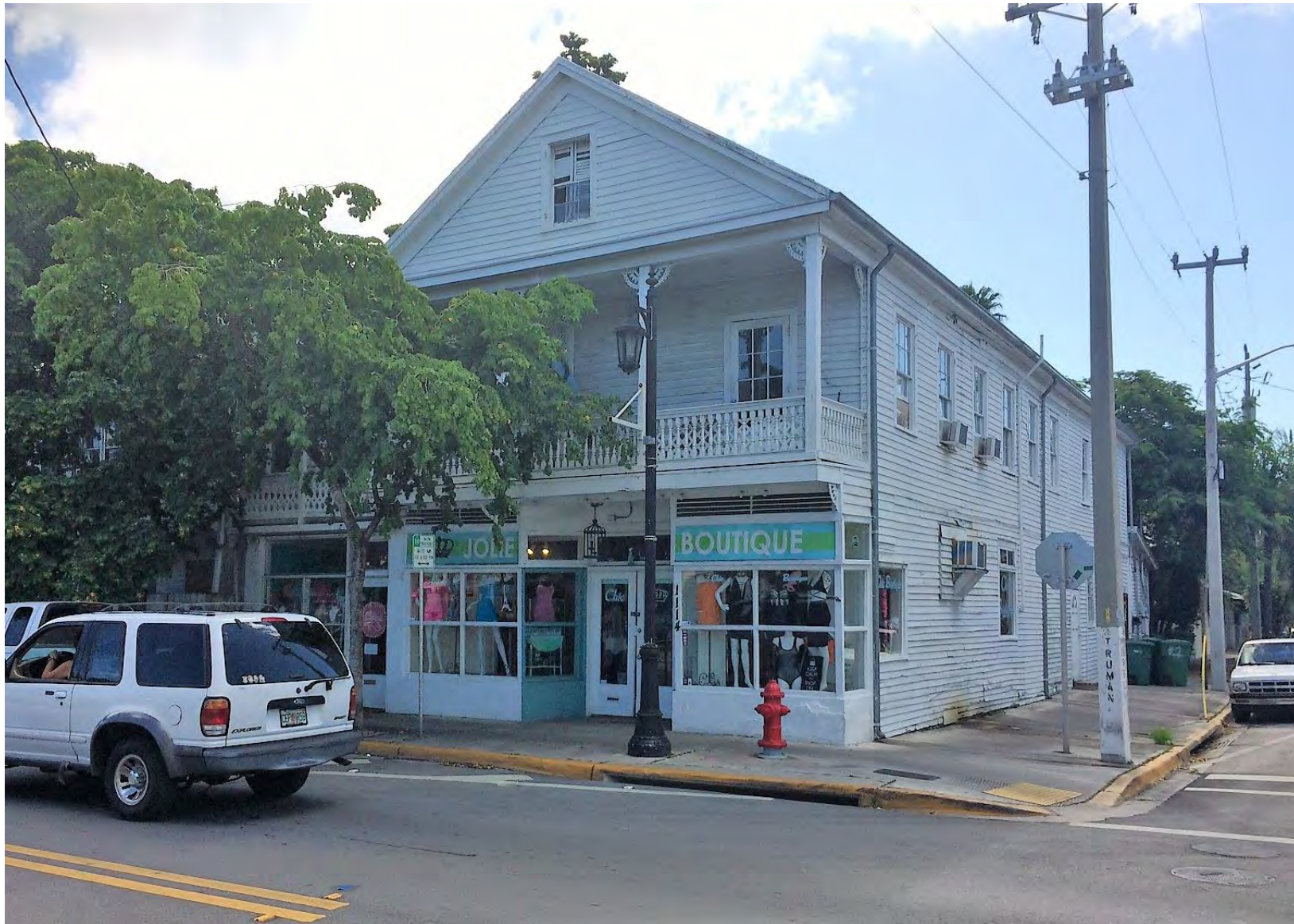
1114 Truman Avenue RIGHT NEIGHBORING PROPERTY FRONT VIEW
