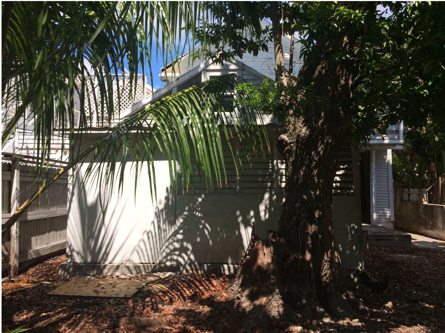
1116 Truman Avenue REAR VIEW
