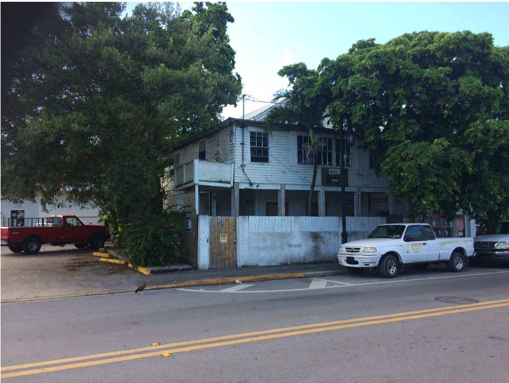
1116 Truman Avenue FRONT VIEW
