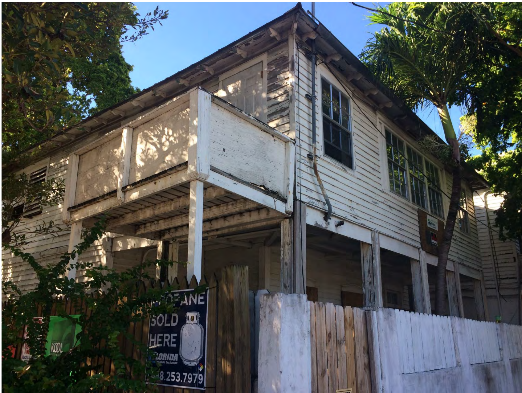
1116 Truman Avenue FRONT VIEW
