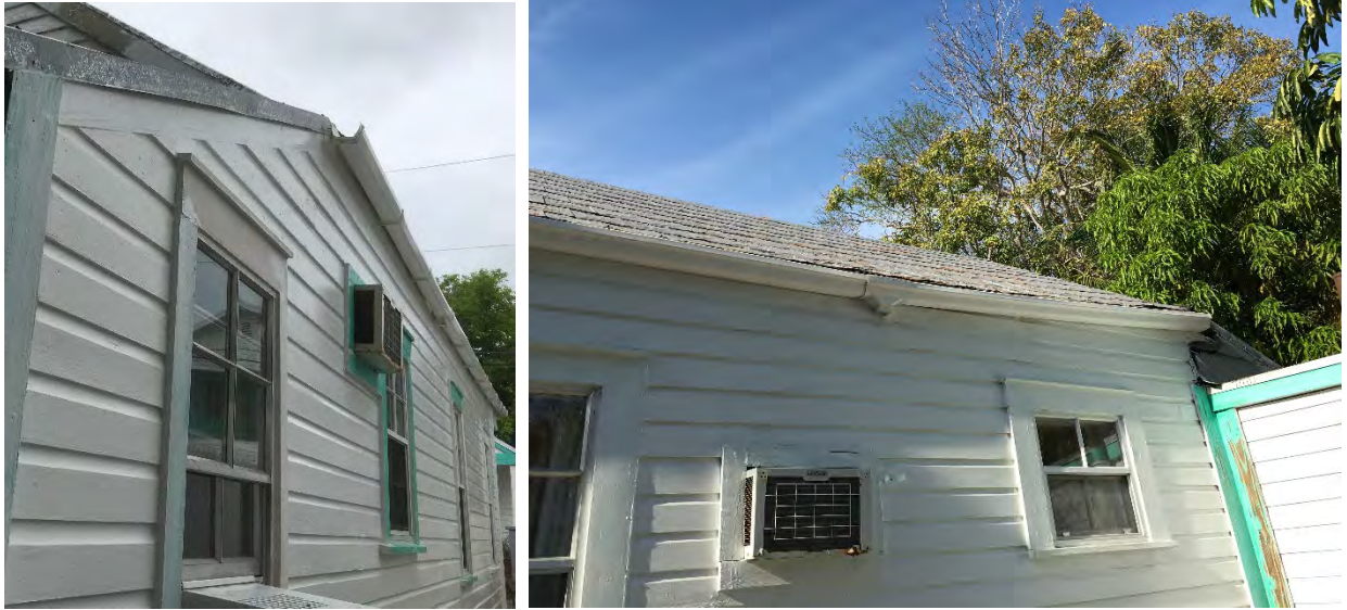
This is the north side of the building Kitchen (south)
