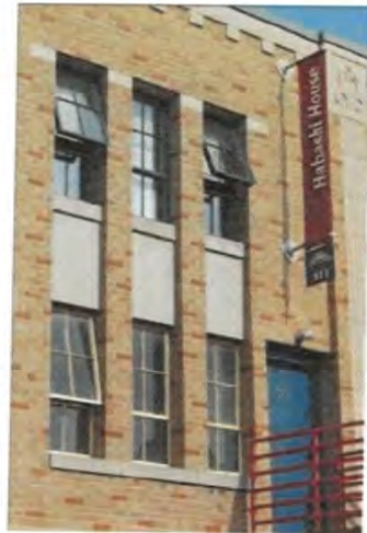
[21] The windows on the lower floor, which were too deteriorated to repair, were replaced with new steel windows matching the upper-floor historic windows that were retained.
