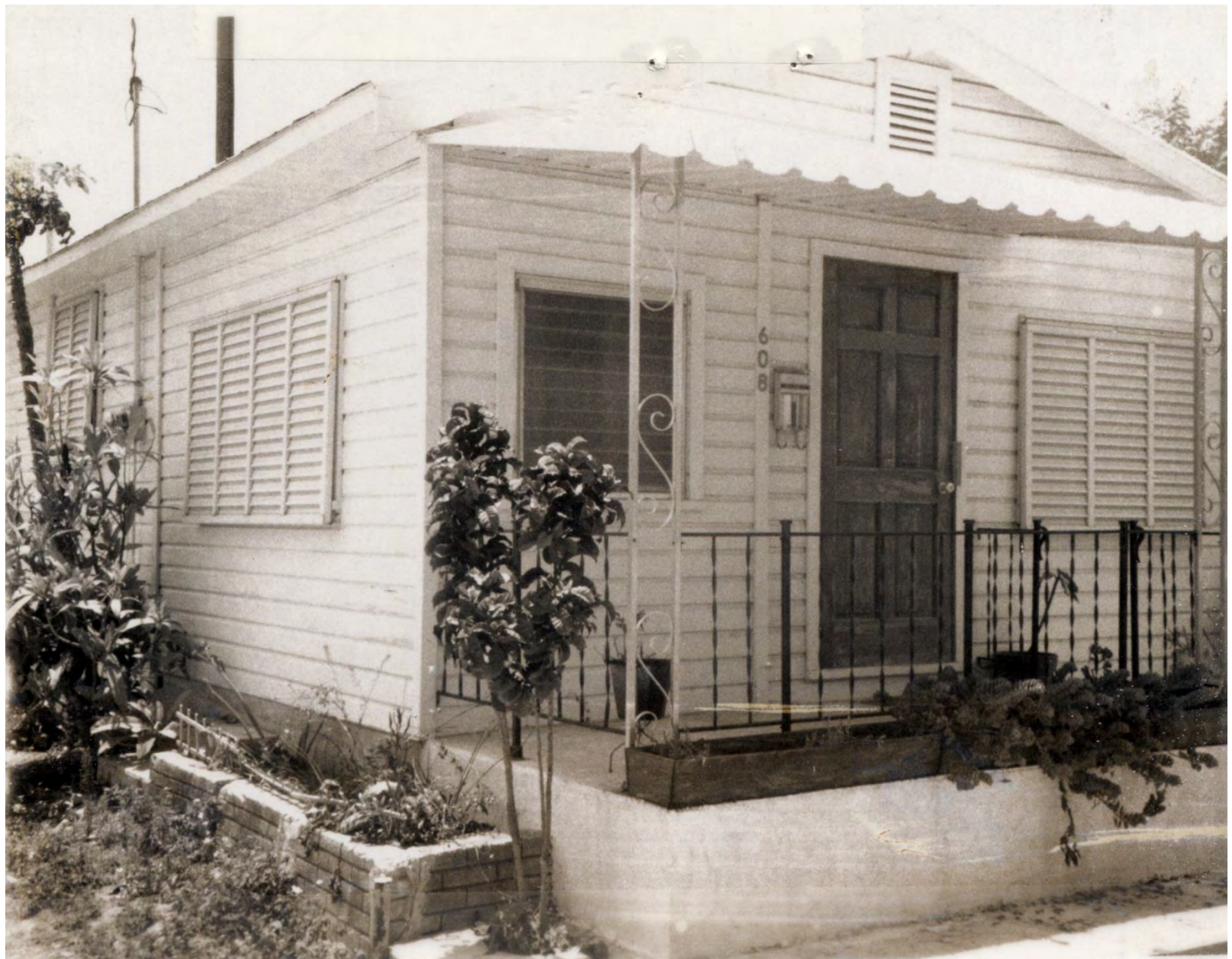
811 Simonton, formerly 608 Petronia Property Appraiser's Photograph, c. 1965. Monroe County Public Library.
