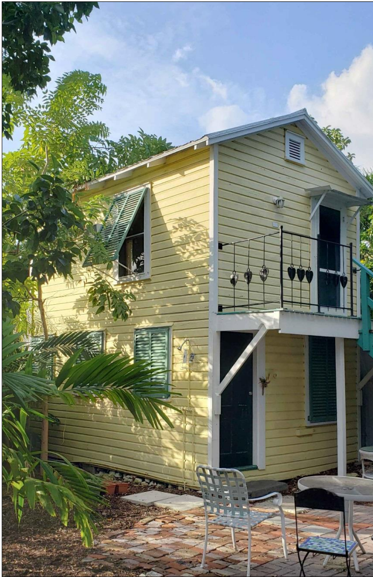
1226 South St, Existing Cottage in Rear Right Corner of the property
