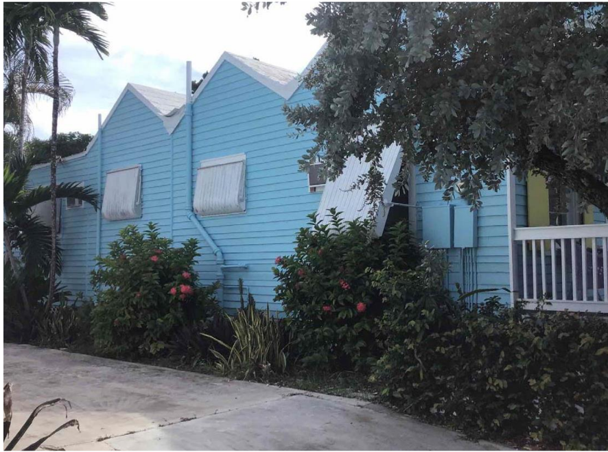
718 Southard Street prior to demolition.
