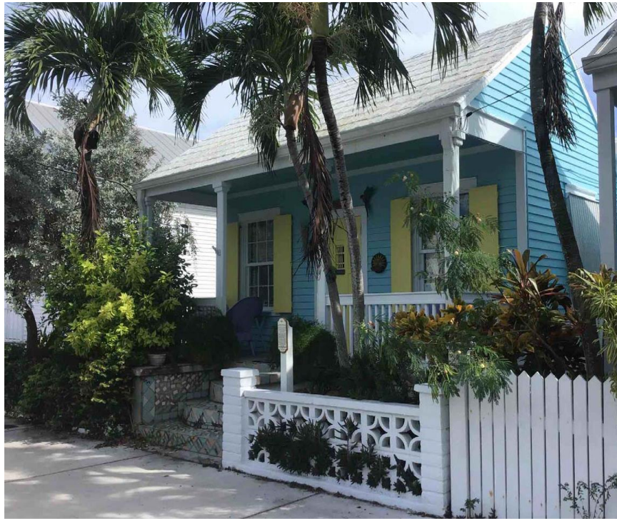
718 Southard Street prior to demolition.
