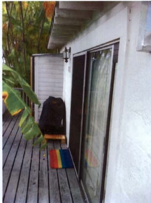
EXISTING REAR DECK TO REMAIN
