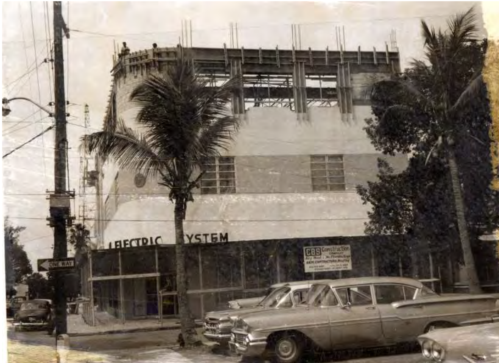
#533 Eaton Street circa 1961 when third floor was under construction. Monroe County Library
