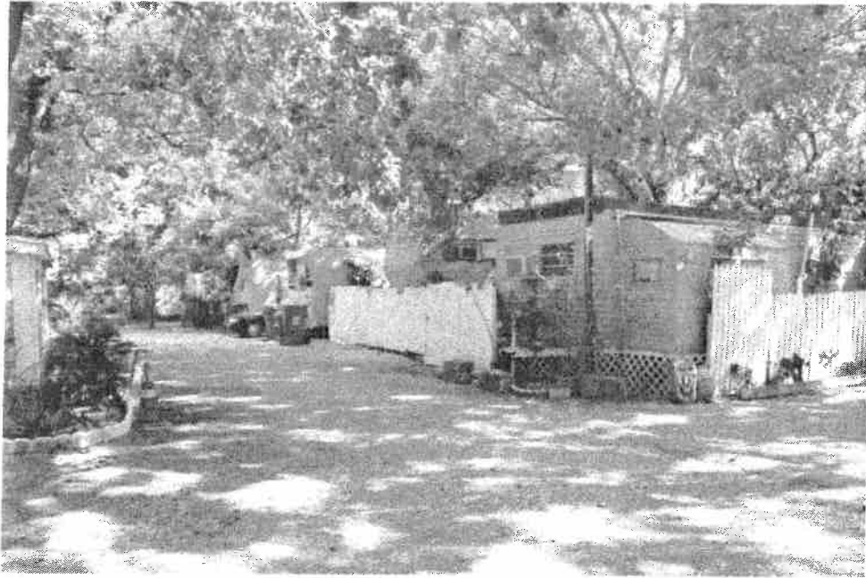
Interior Lane Looking From Unit 29 to 23 (Entry Driveway is on the Right):
