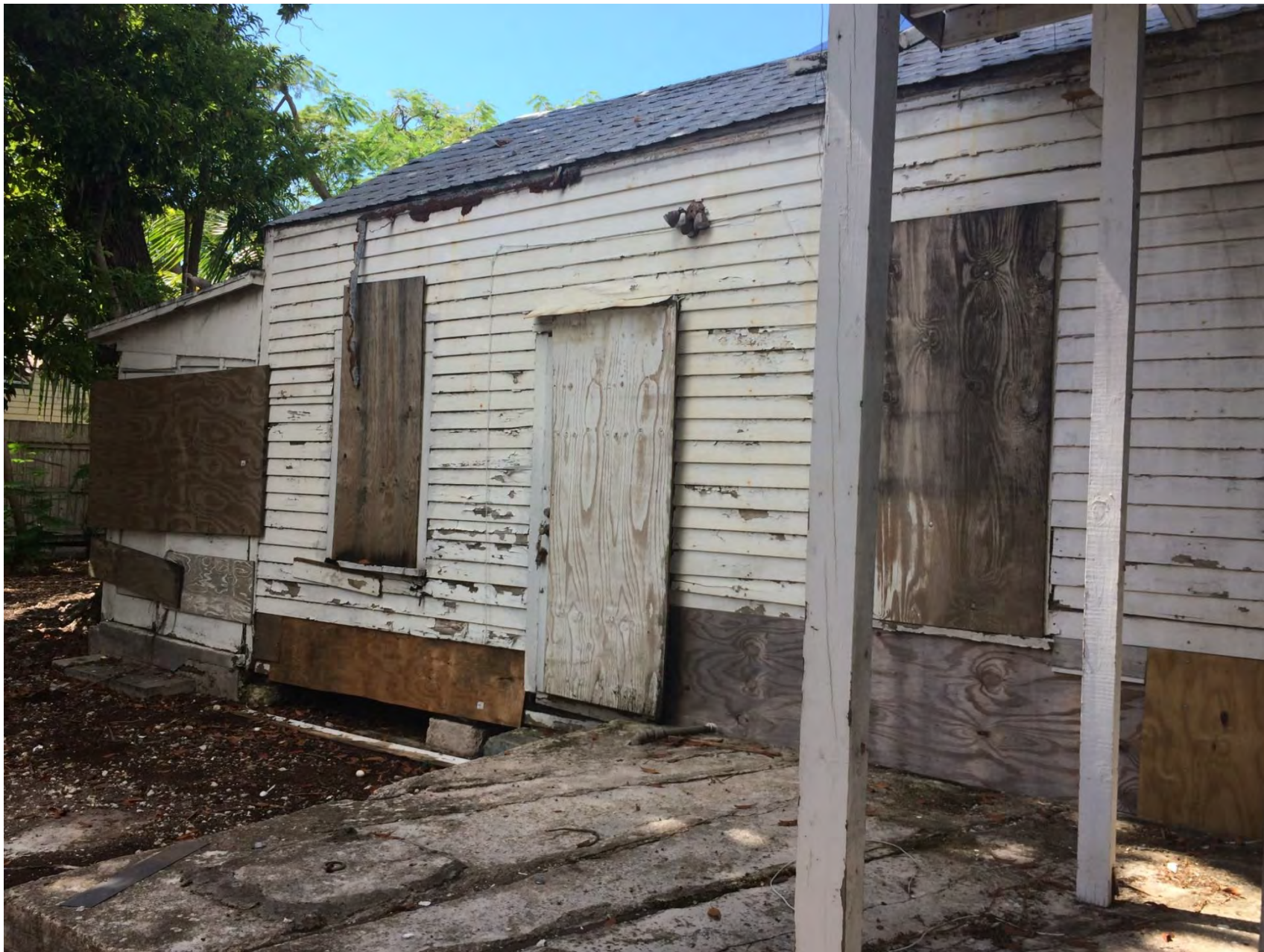
1116 Truman Avenue PARTIAL SIDE VIEW
