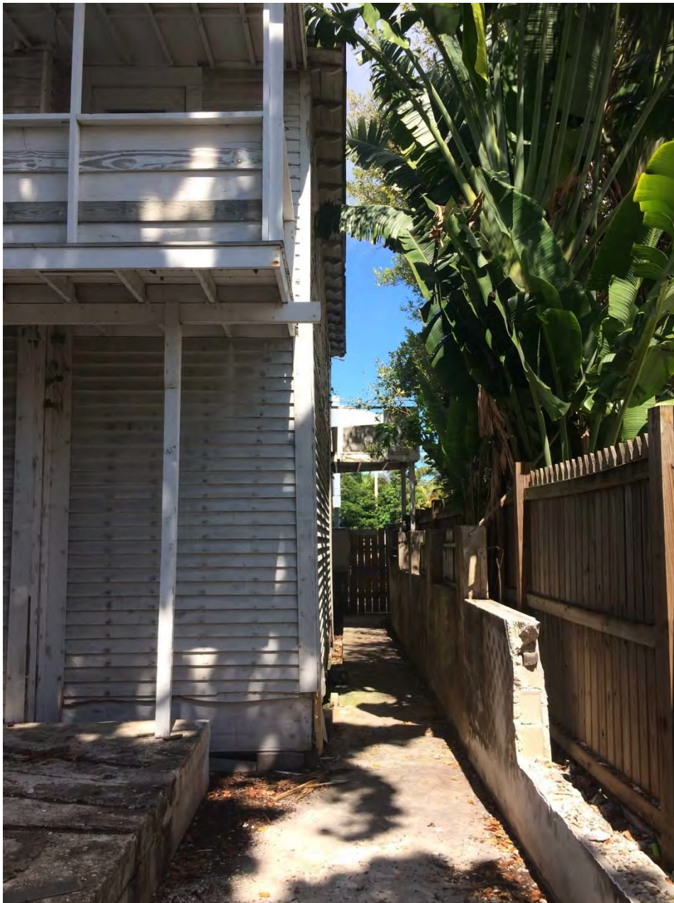
1116 Truman Avenue PARTIAL SIDE VIEW
