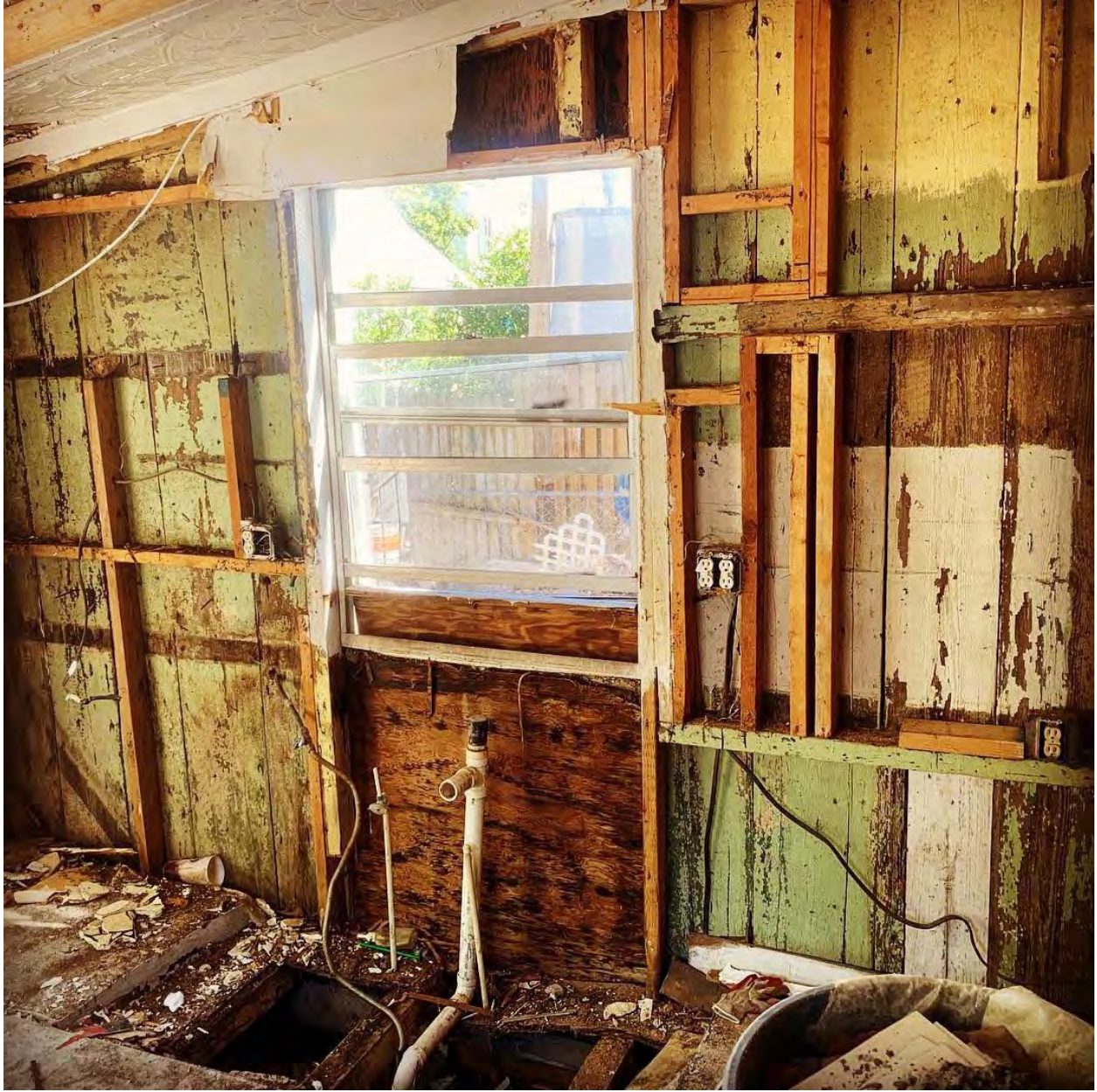
INSIDE OF REAR ADDITION (TO BE REMOVED)
