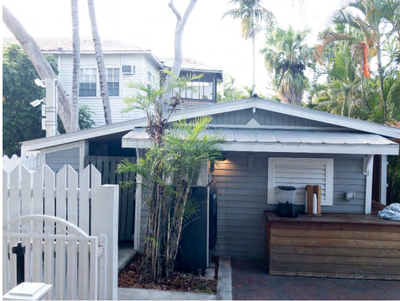
VIEW DUE NORTH – The structure faces the rear of Chelsea, with a pool deck on the right, and parking lot on the left. The Poinciana trees can be seen on the rear left.
