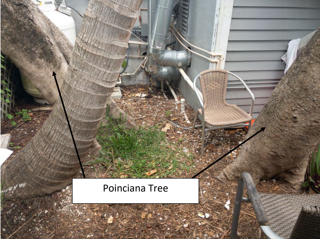
VIEW NORTHWEST CORNER OF LAUNDRY – The two tree bases of the Poinciana trees.
