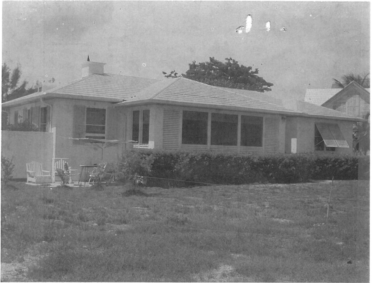
Photo taken by the Property Appraiser's office c1965; 400 South St.; Monroe County Library
