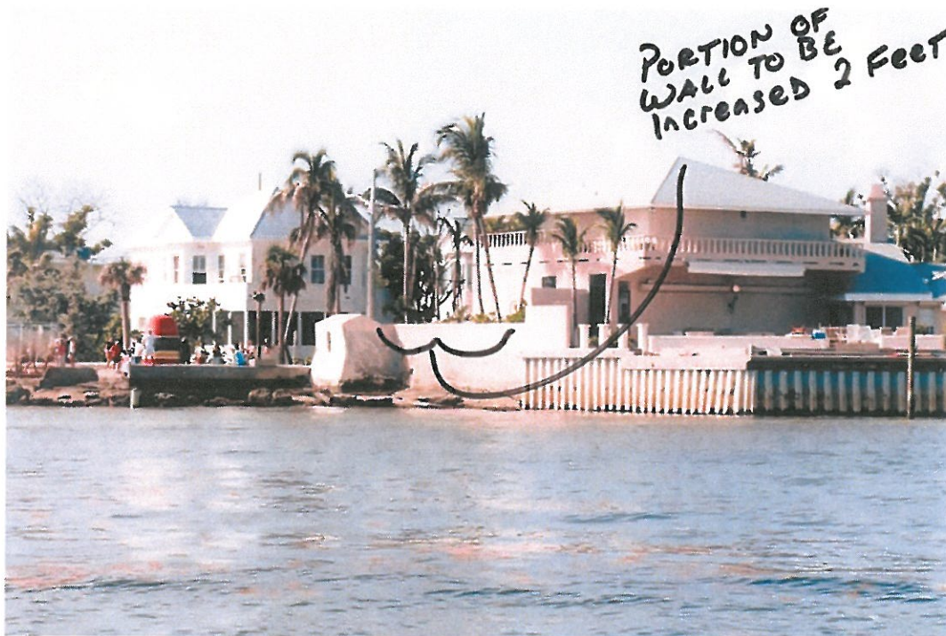
Photo 1 - View looking North towards the subject property, from Atlantic Ocean, denoting the portion of the wall which applicant requests to increase.
