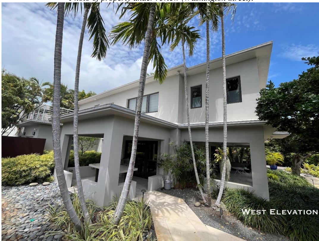
Photo of property under review (West Elevation).
