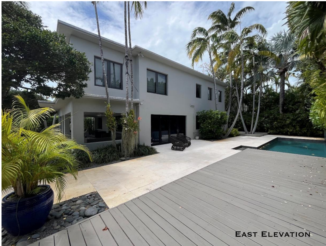
Photo of property under review (East Elevation).
