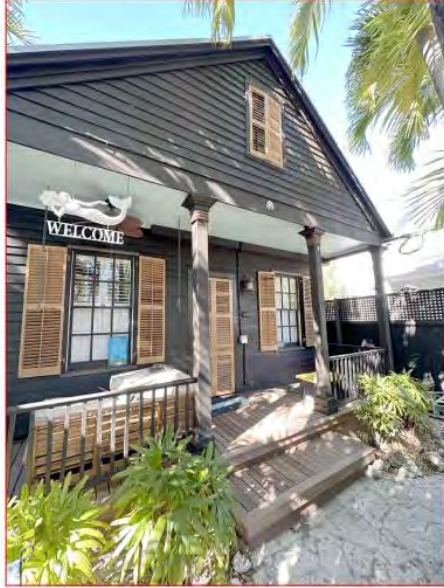
Existing Front of Historic Structure
