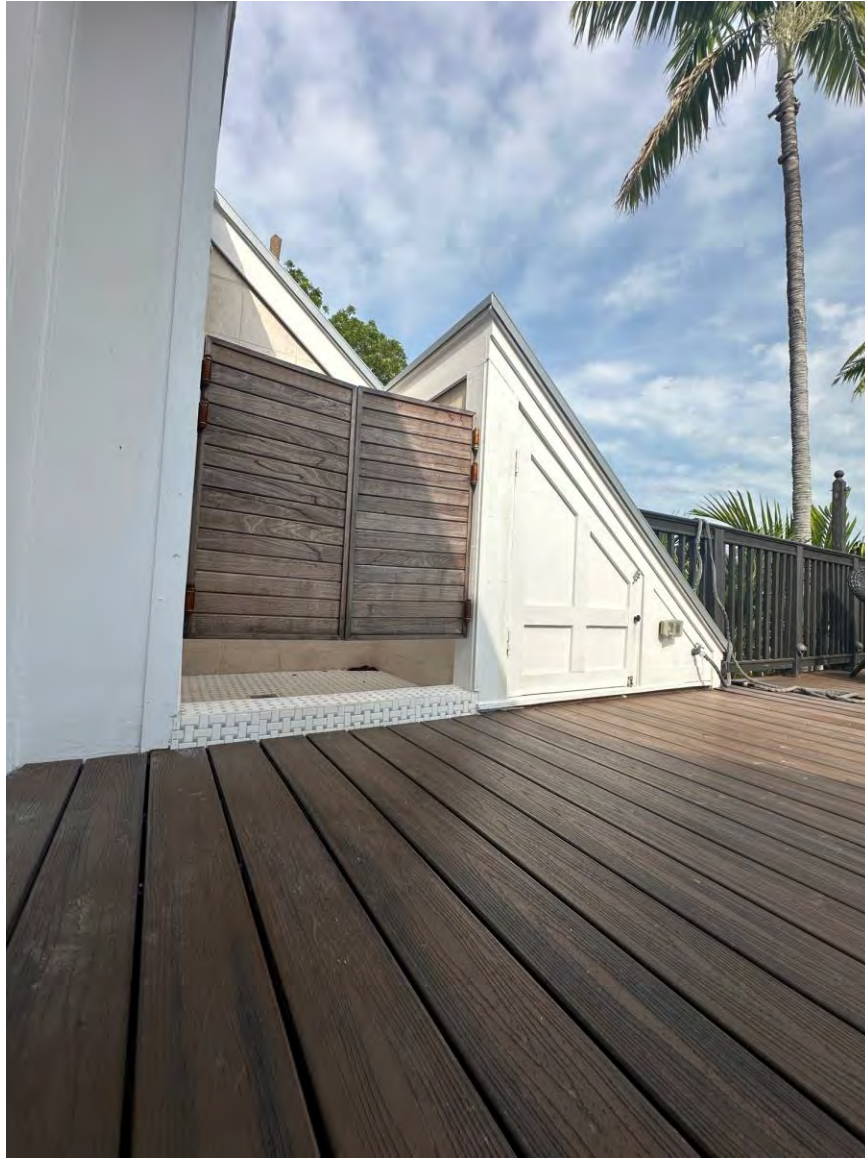
Roof Deck Existing Conditions
