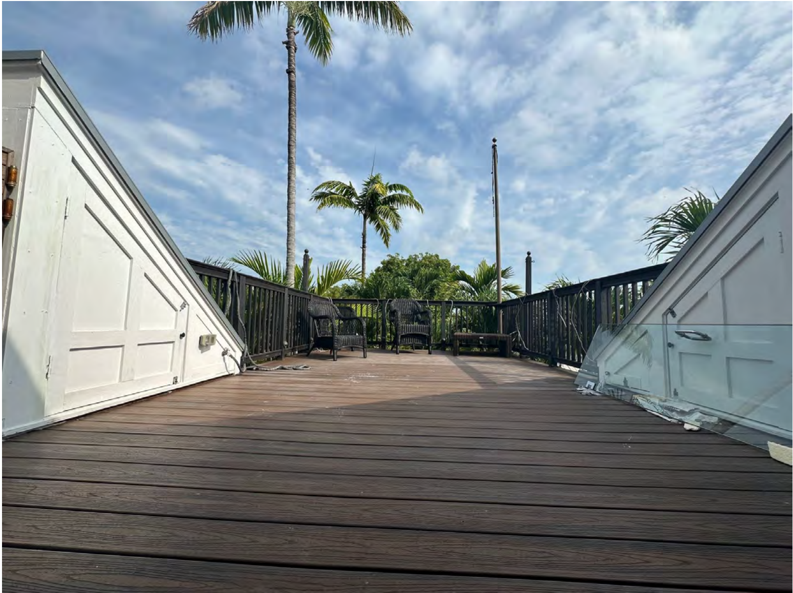
Roof Deck Existing Conditions
