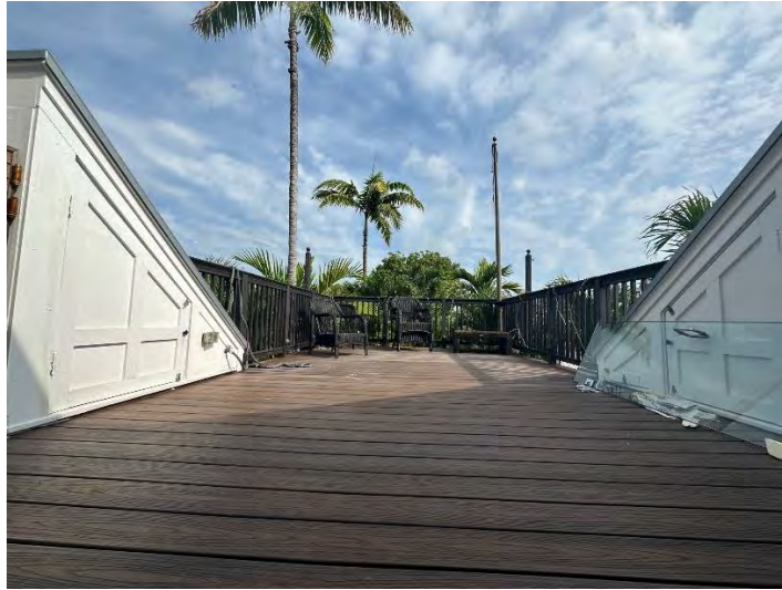
Existing Roof Deck Conditions
