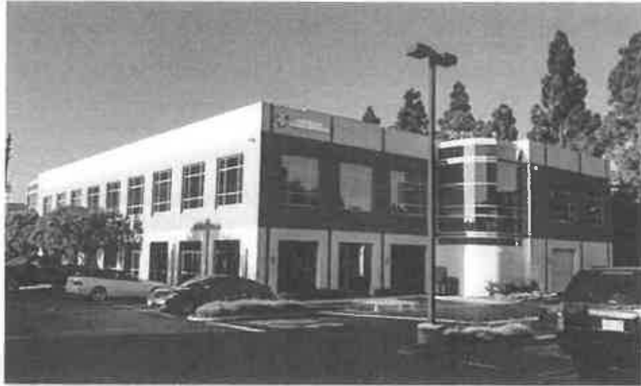
Pictured above: AGS Headquarters in Los Angeles, CA.
