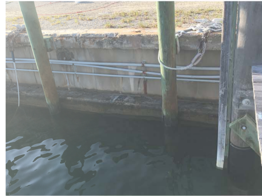
FIGURE 106-A: VIEW OF EXISTING SEAWALL EAST OF DOCK 2
