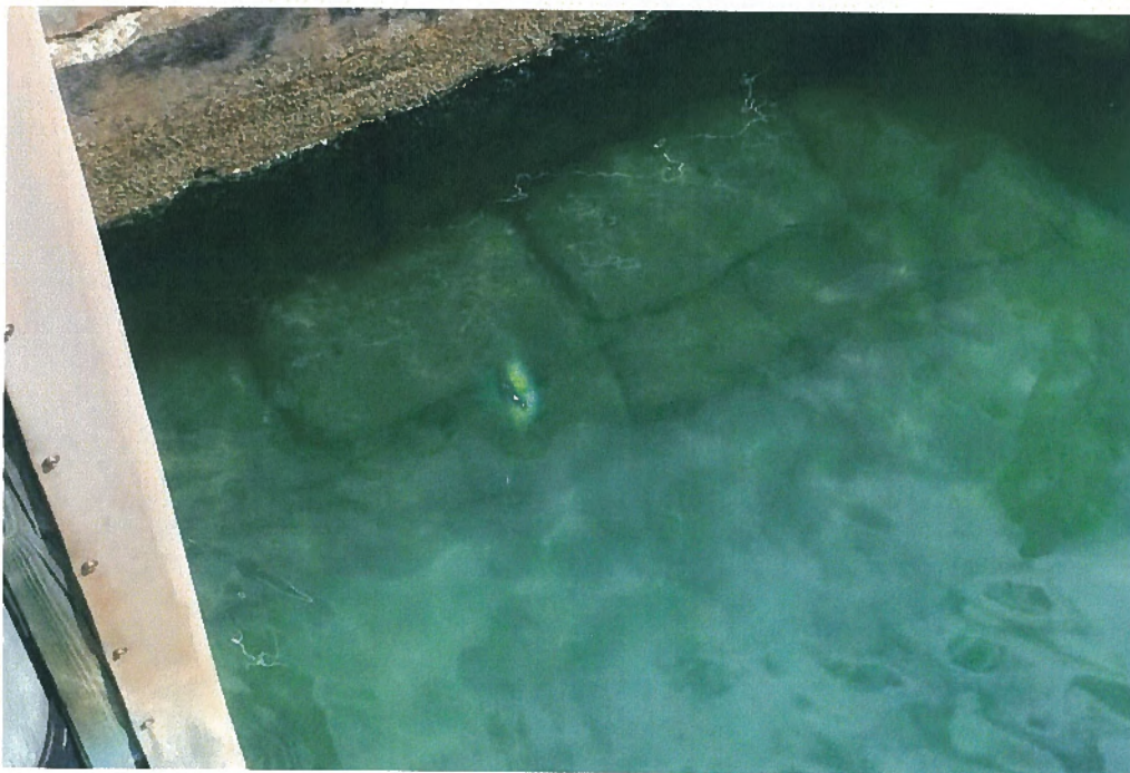
4) Sand-Cement Bags by Toe of Seawall
