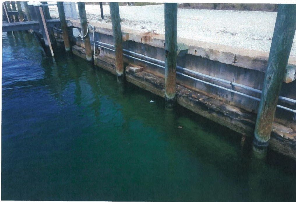
2) Typical View of Existing Seawall
