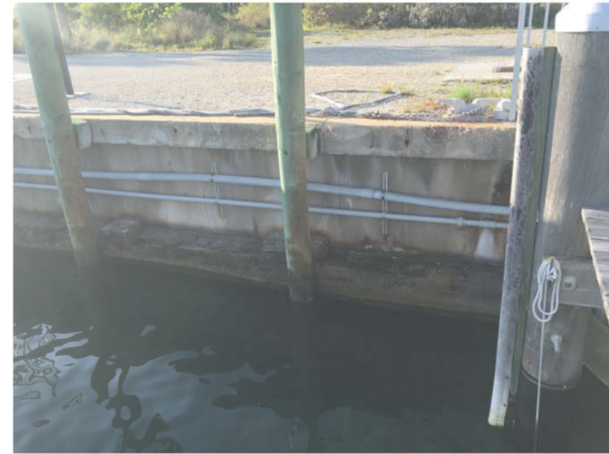
FIGURE 108-A: VIEW OF EXISTING SEAWALL EAST OF DOCK 4
