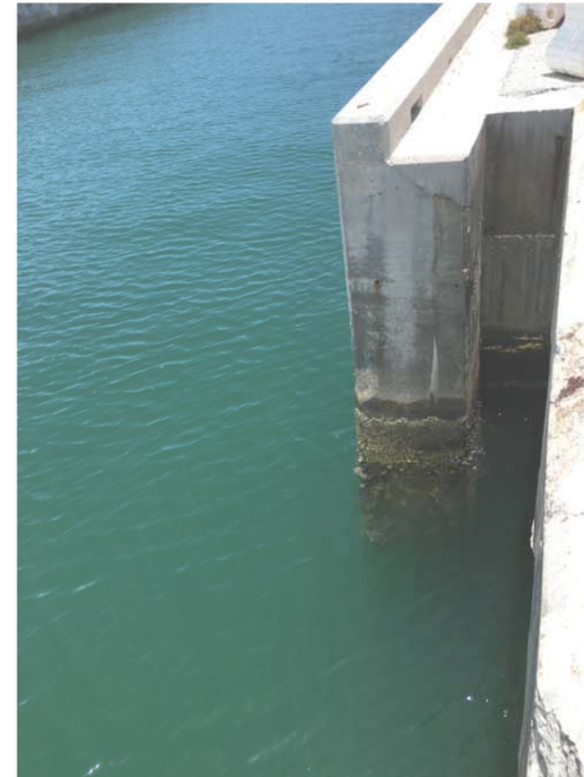
FIGURE 110-A: VIEW OF EXISTING SEAWALL EAST OF TRIANGLE
