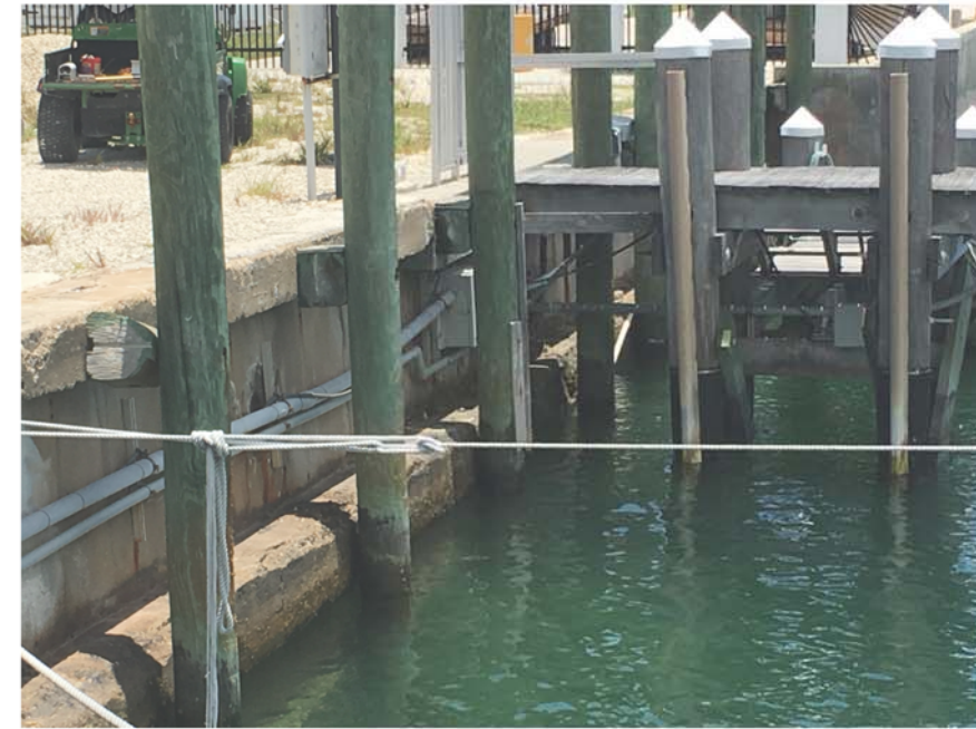
FIGURE 109-A: VIEW OF EXISTING SEAWALL EAST OF DOCK 5
