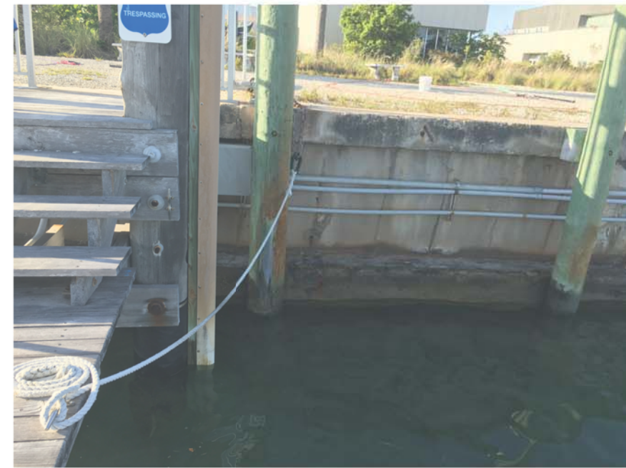
FIGURE 105-B: VIEW OF EXISTING SEAWALL WEST OF DOCK 1
