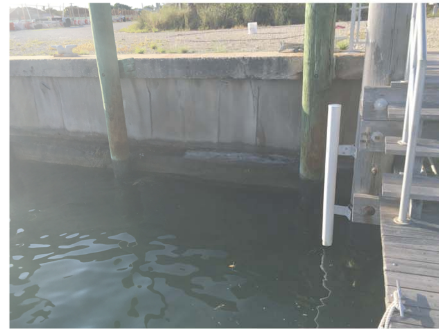
FIGURE 105-A: VIEW OF EXISTING SEAWALL EAST OF DOCK 1
