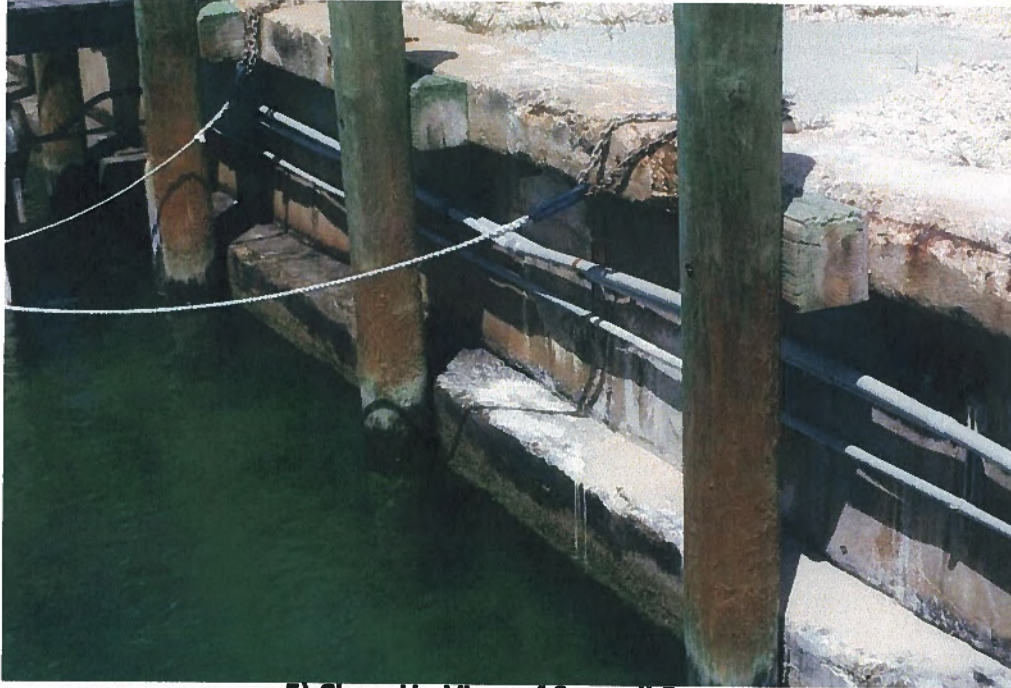
5) Close-Up View of Seawall Front
