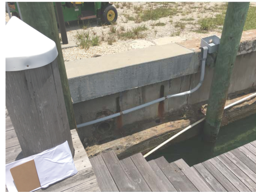
FIGURE 109-B: VIEW OF EXISTING SEAWALL WEST OF DOCK 5
