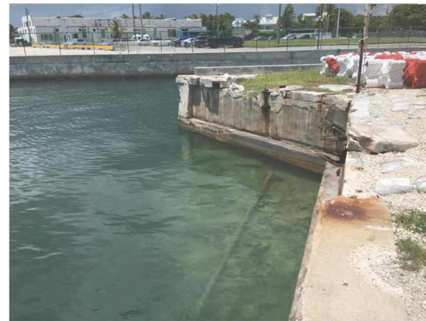
FIGURE 110-B: VIEW OF EXISTING SEAWALL WEST OF TRIANGLE
