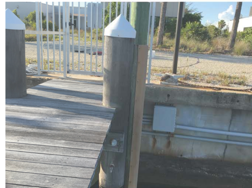
FIGURE 106-B: VIEW OF EXISTING SEAWALL WEST OF DOCK 2
