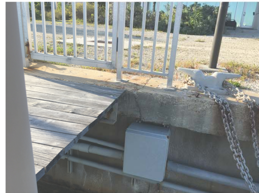
FIGURE 108-B: VIEW OF EXISTING SEAWALL WEST OF DOCK 4
