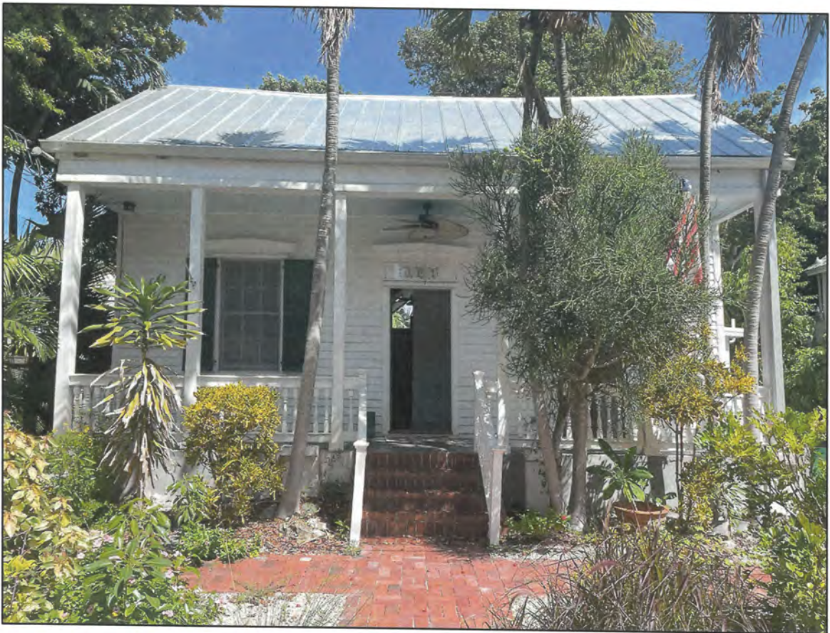
VIEW FROM CATHOLIC LANE (EXISTING WEST ELEVATION)
