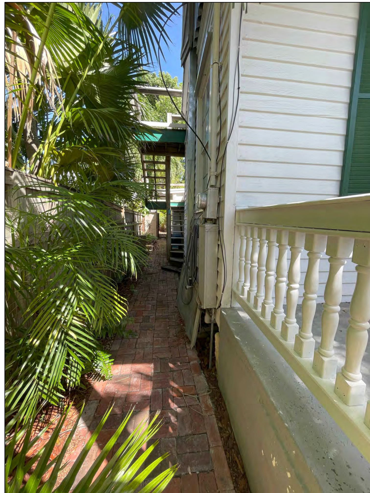
2 A8 VIEW FROM SIDE OF THE HOUSE (EXISTING NORTH ELEVATION) SCALE: N.T.S.
