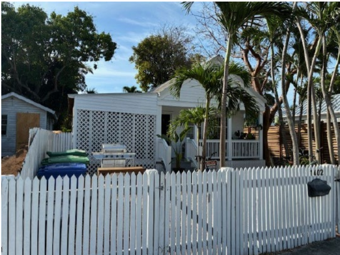
Front of Property Under Review.
