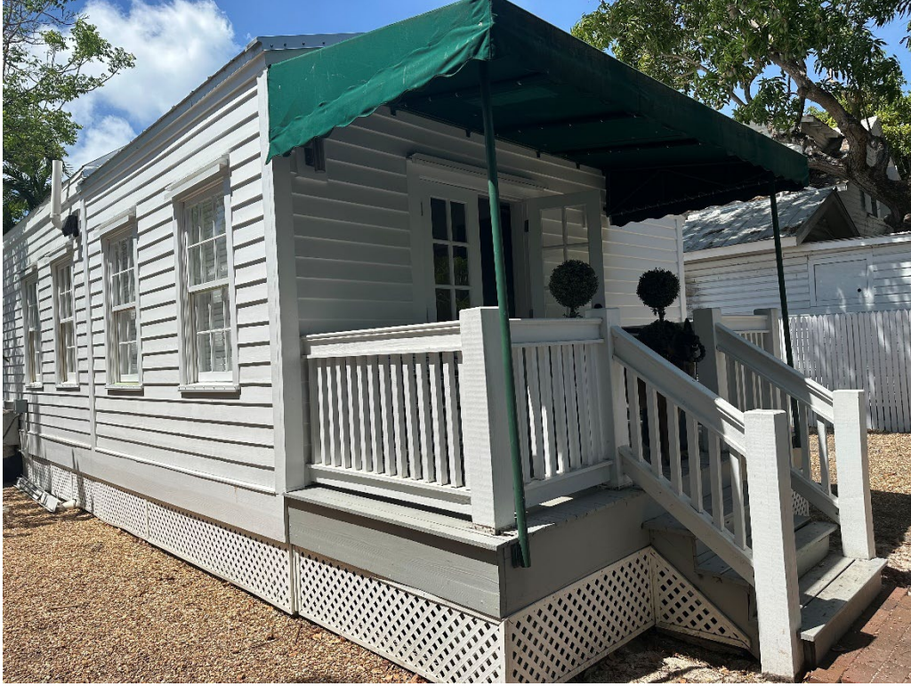
View of Rear of Property Under Review.
