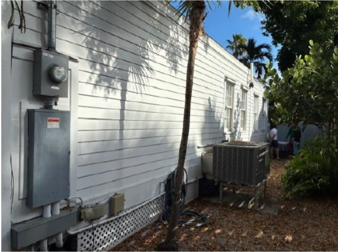
View of West Elevation of Property Under Review.
