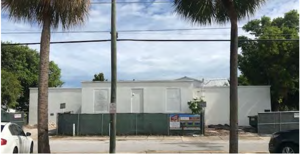
Current Front Street Façade.
