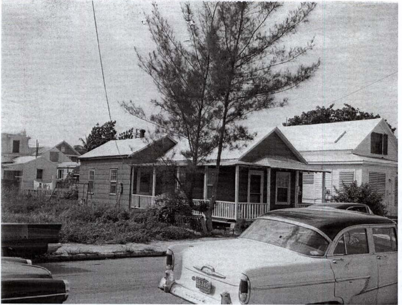
Photo taken by Property Appraiser's office c1965; 914 James St. Monroe County Library
