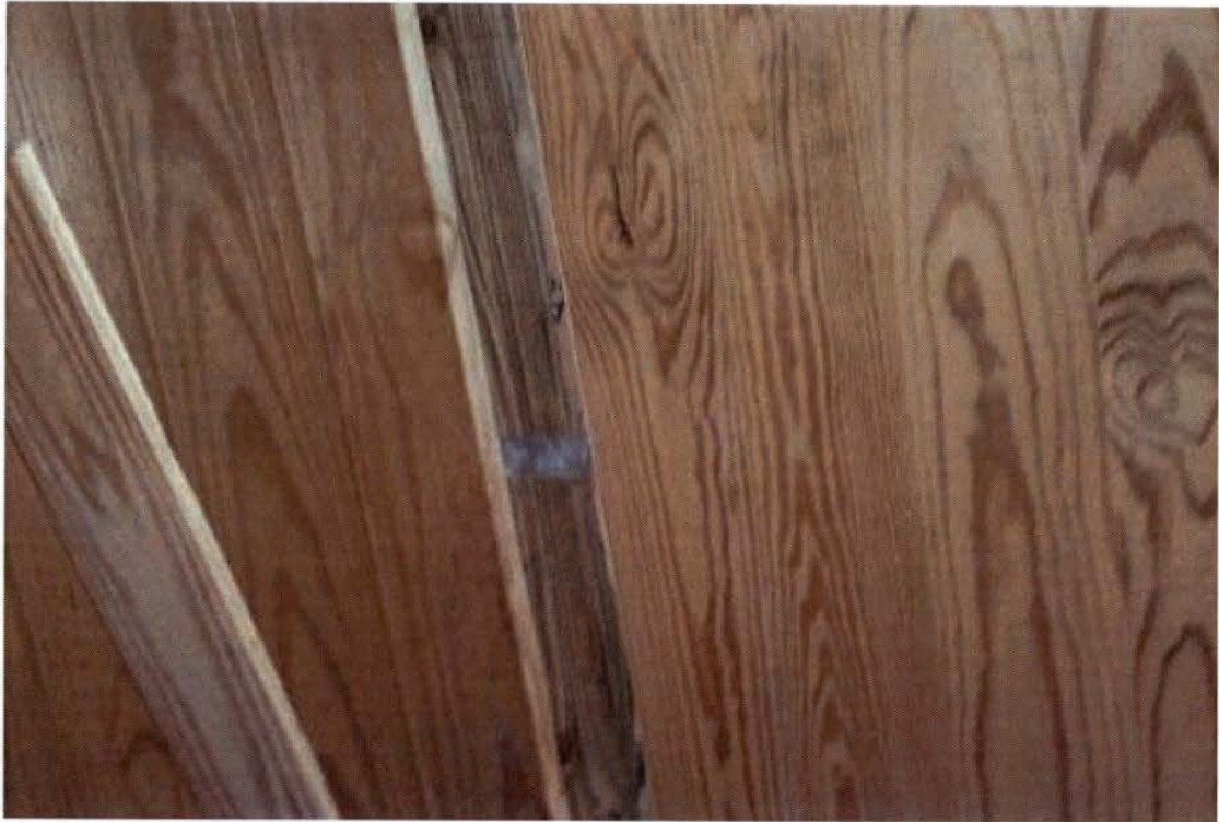
NEW WOOD FRAMING & STRAPPING @ EXISTING NON-HISTORIC REAR ADDTION
