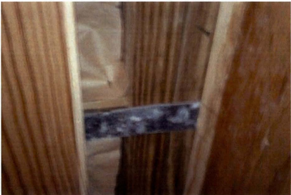
NEW WOOD FRAMING & STRAPPING @ EXISTING NON-HISTORIC REAR ADDITION
