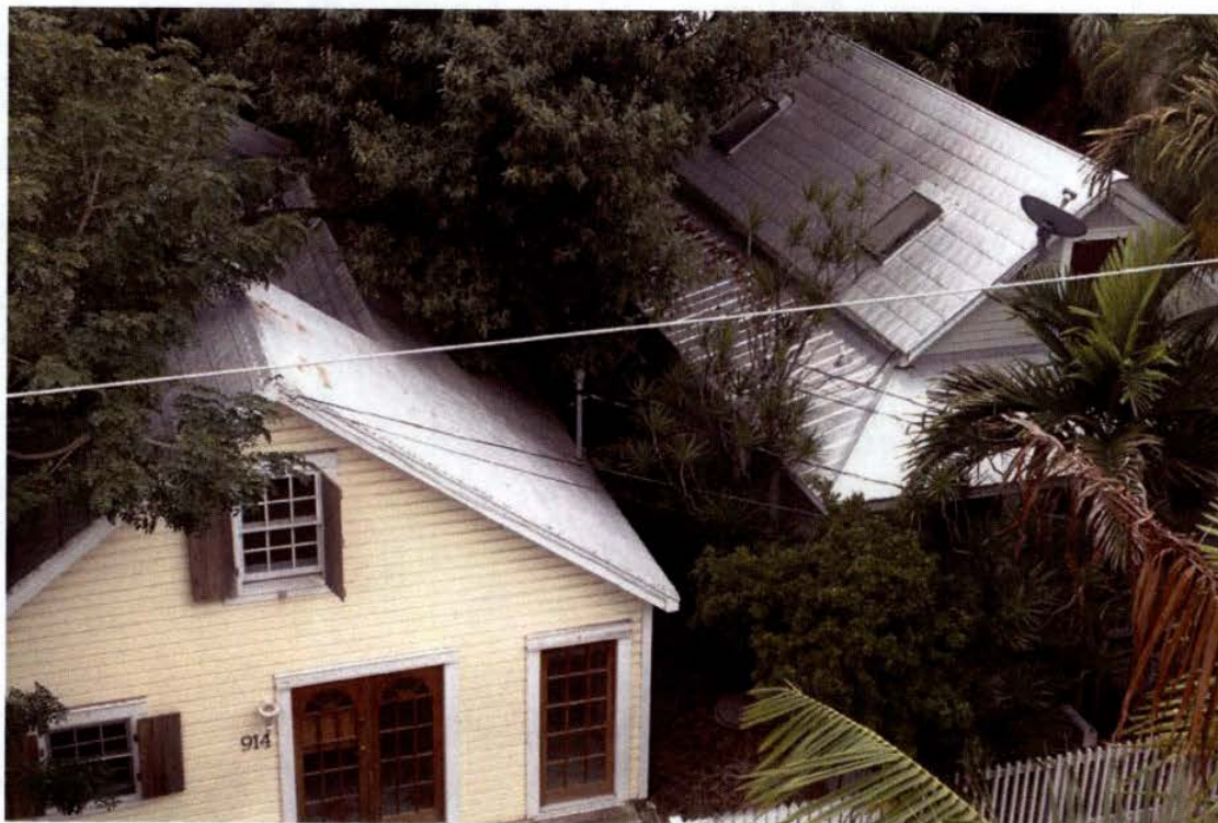
FRONT ELEVATION & NEIGHBORING STRUCTURE
